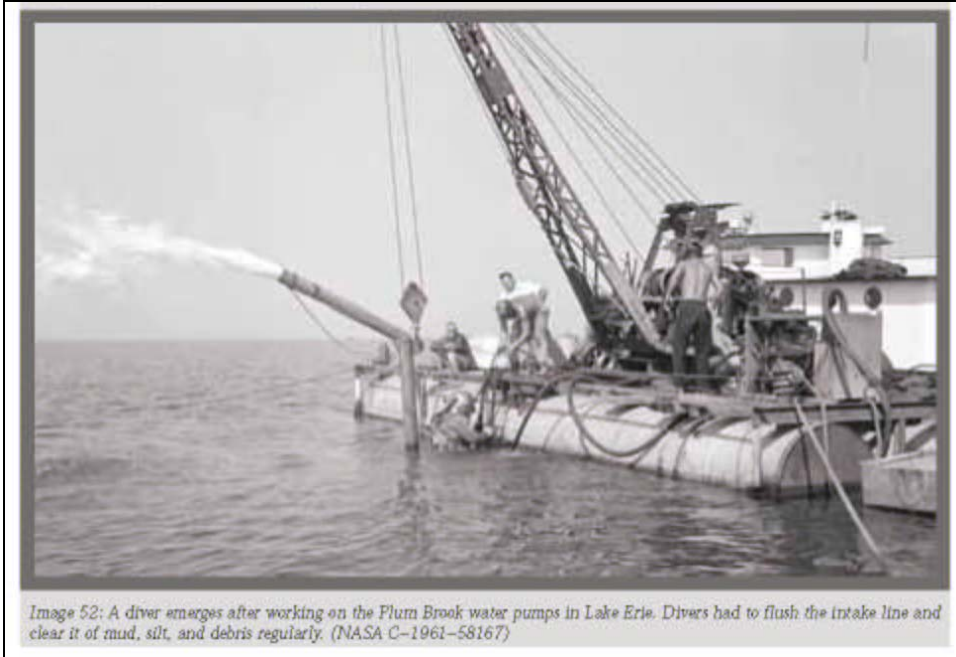
Figure 7. Maintenance work to clear silt and debris from water intake. NASA photograph dated 1961 (from Bowles and Arrighi (2004), Image 52)
