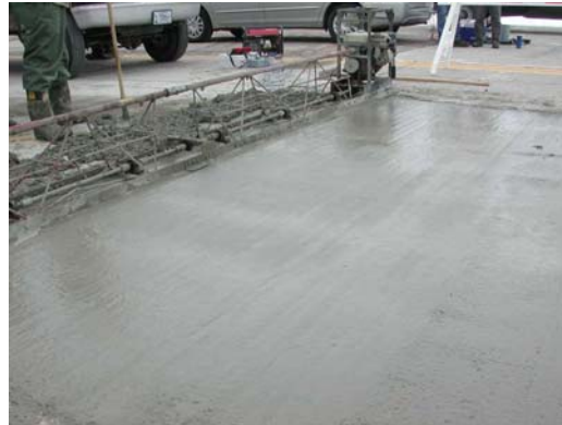
Figure 5. Screeding the top layer of concrete.
