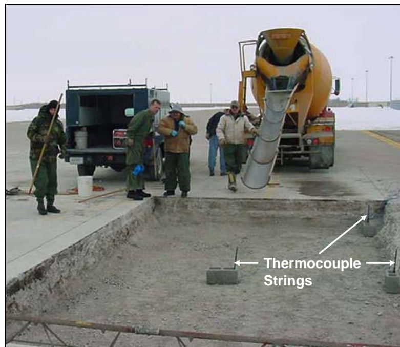
Figure 2. Repair section instrumented with thermocouples.
