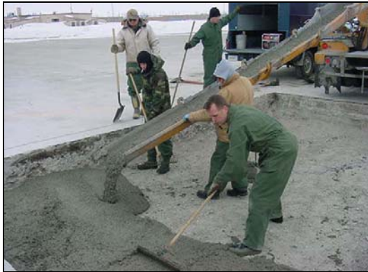
Figure 4. Placing and raking intermediate layers of concrete.
