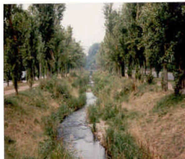
Figure 1. Low-flow channels can maintain natural stream characteristics within an enlarged floodway
