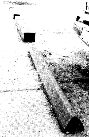
Plastic wheel stop with wood crosstie wheel stops in background
