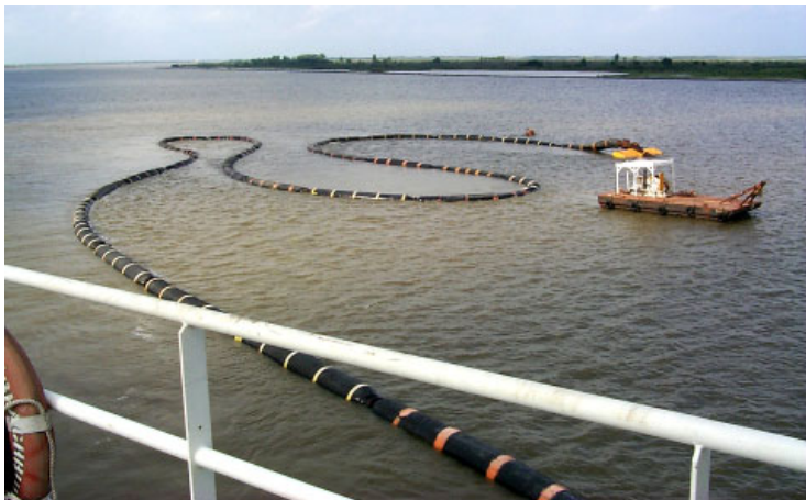
Figure 5. Anchor barge (skidder) holding floating hose and hard point
