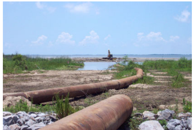
Figure 6. Shore pipe with marsh buggy in background
