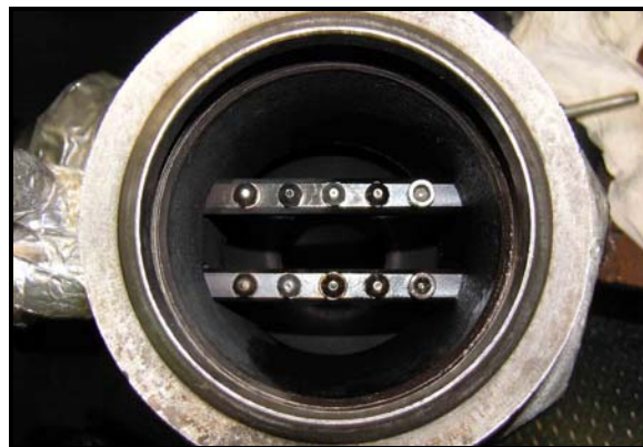
Figure 17. Upstream view into the fill air manifold of the fuel inlet manifold with spray bars Delavan fuel flow nozzles
