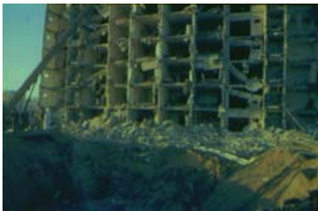
Fig. 24-1. Remains of Khobar Towers in Dhahran, Saudi Arabia. On 25 June 1996, terrorists bombed this complex, which was used as a barracks for US Air Force personnel. Note the large crater in front of the building and the loss of the building closest to where the truck bomb was parked. This bombing caused 19 deaths and 500 injuries.
