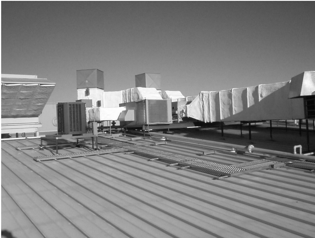
Figure 34. Rooftop view of air conditioners, walkways, and spray-on insulation.
