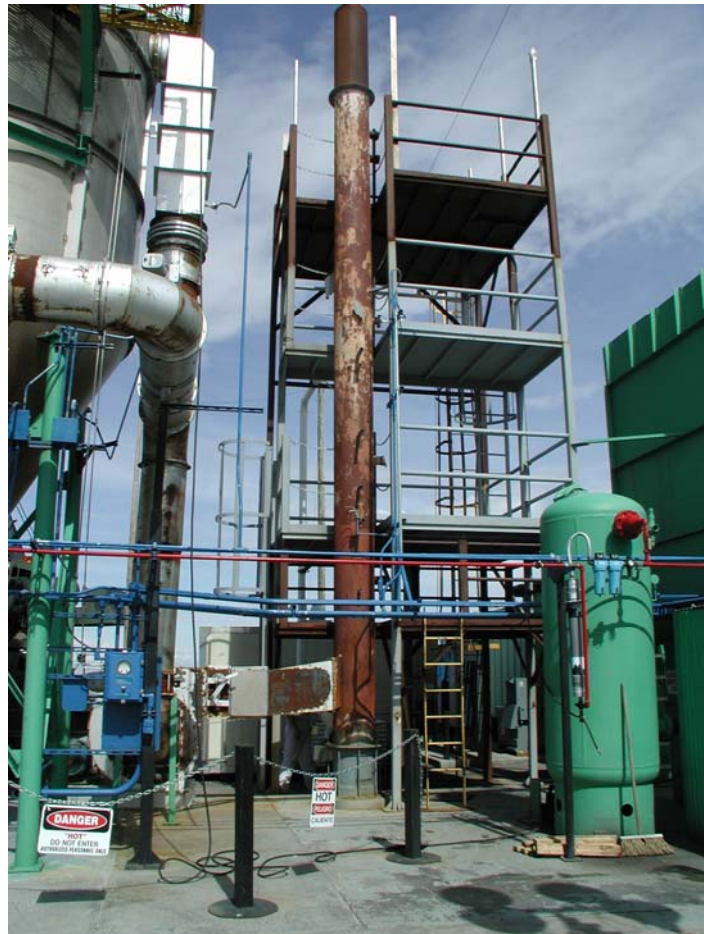
Figure 3-2. TEAD Incinerator Stack.
