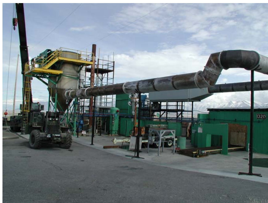
Figure 3-1. TEAD Deactivation Incinerator Building 1320.
