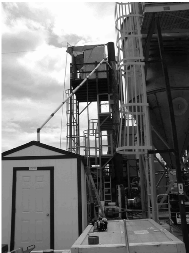
Figure 4. XCEM housing and transport line, M29 sampling setup, stack, and ceramic baghouse at TEAD.
