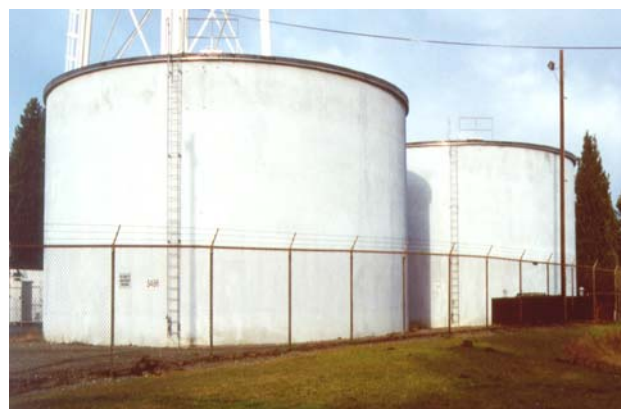
Figure 12. Concrete water tanks reinforced with FRP at Fort Lewis, WA.
