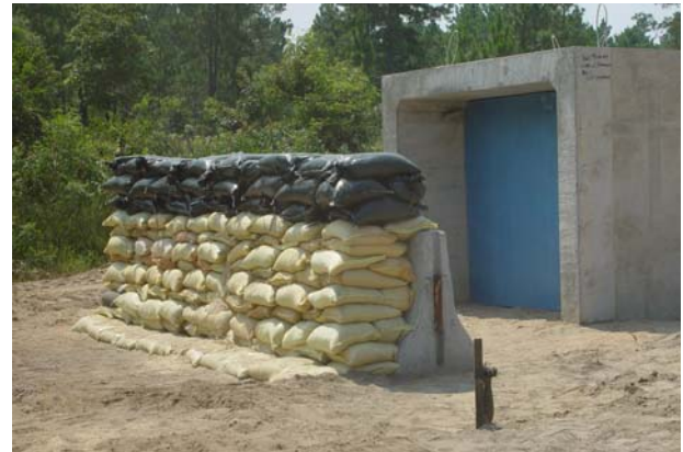
Figure 12. Round 1 placed outside "SCUD bunker"
