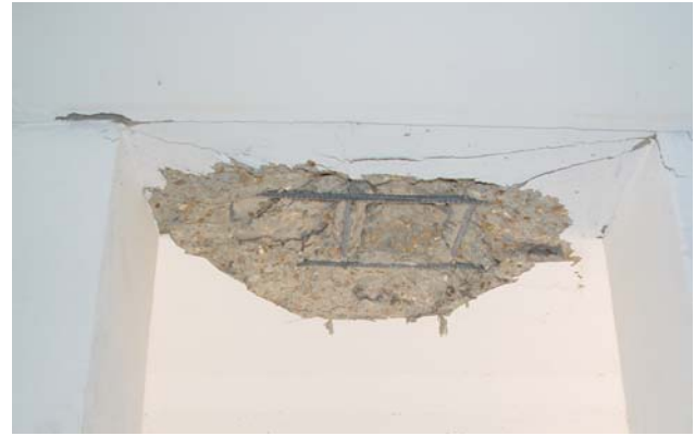
Figure 15. Internal spall surface from Round 1
