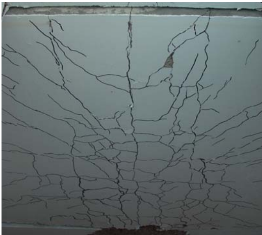
Figure 16. Internal damage from Round 2
