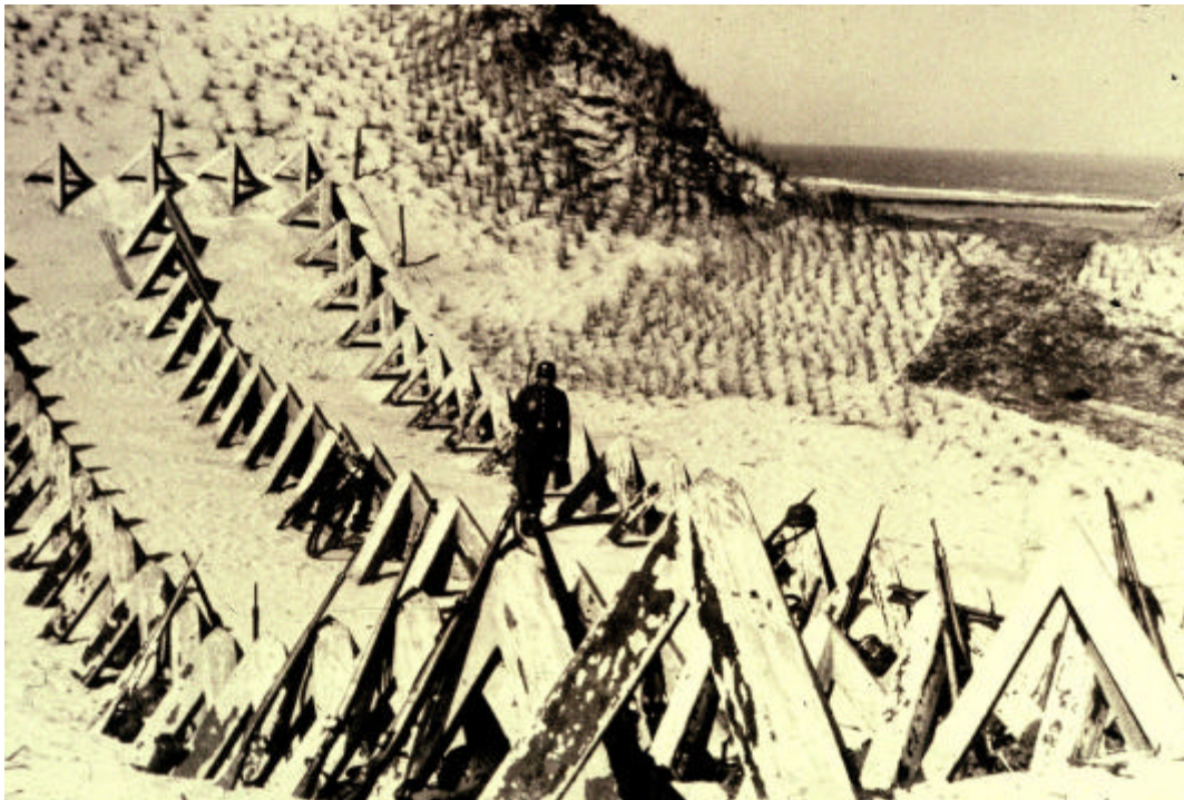
Fig. 11. German obstacle belt covering Normandy beach exit. Reprinted courtesy of CARL.
