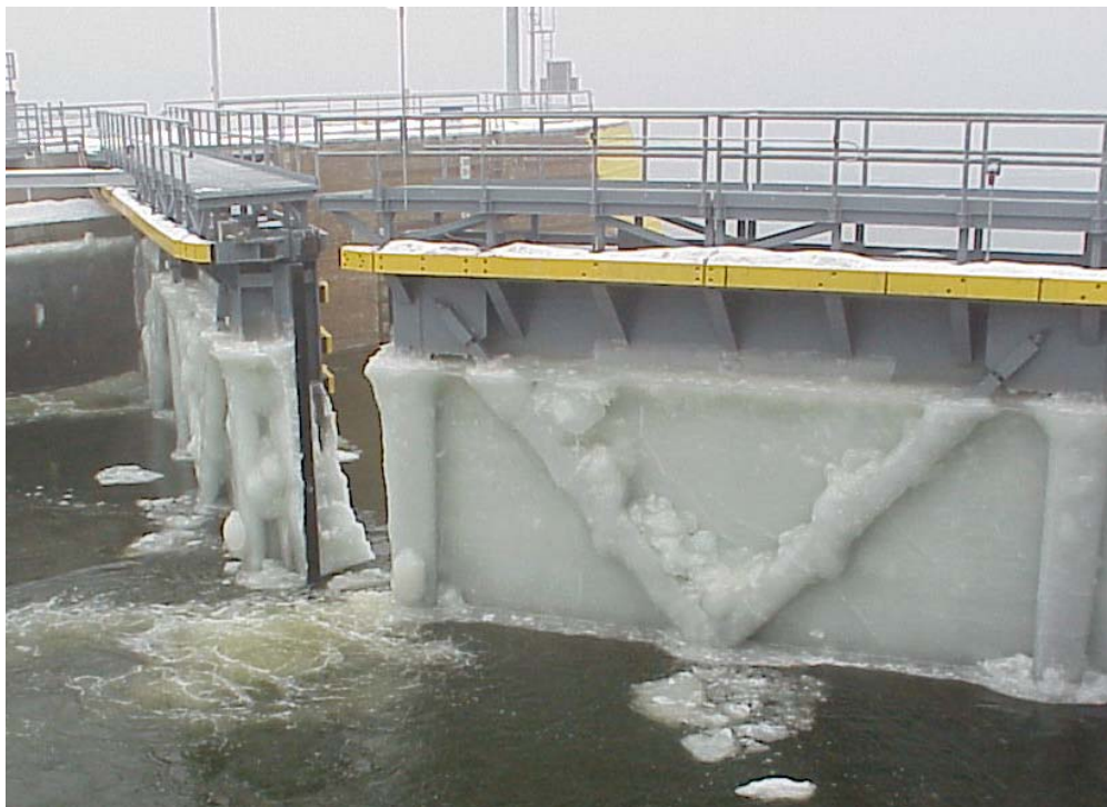
Figure 1. Ice buildup on miter gate at a Mississippi River navigation lock.
