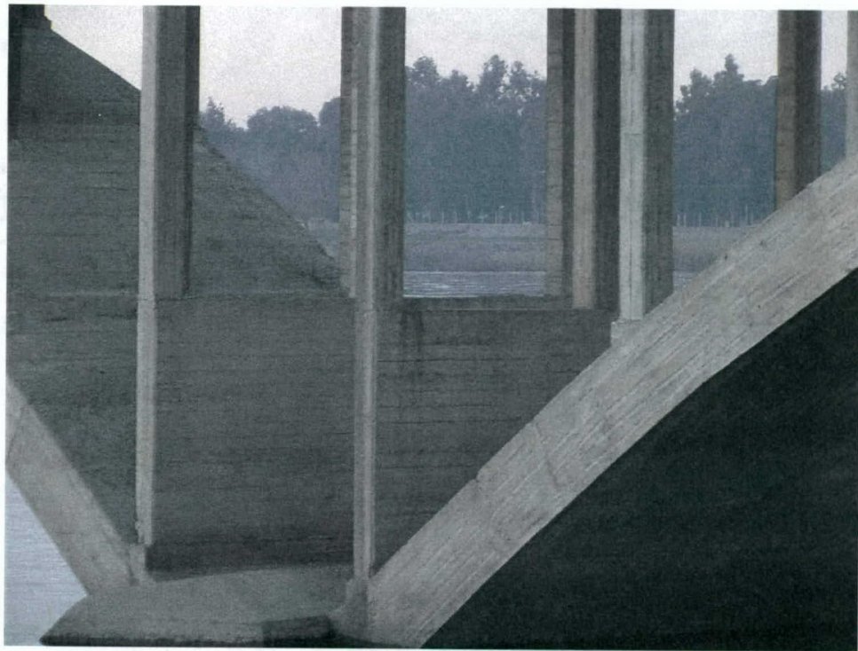
Figure D9. The arches, and the column wall of the Birecik Bridge
