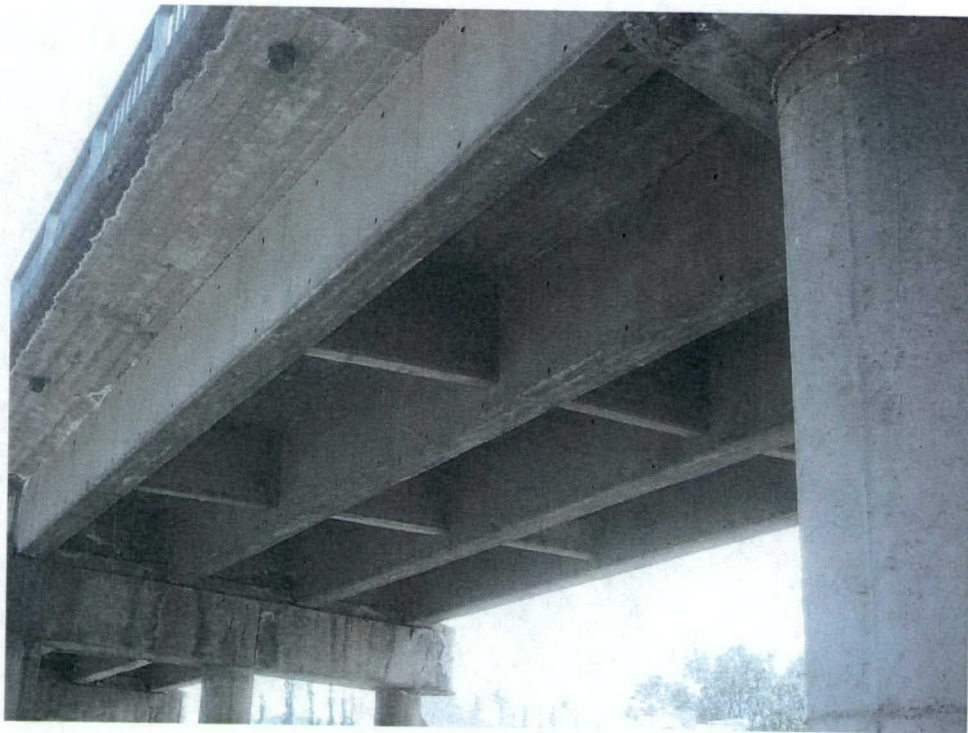
Figure E7. The exterior girder of the Candir Bridge
