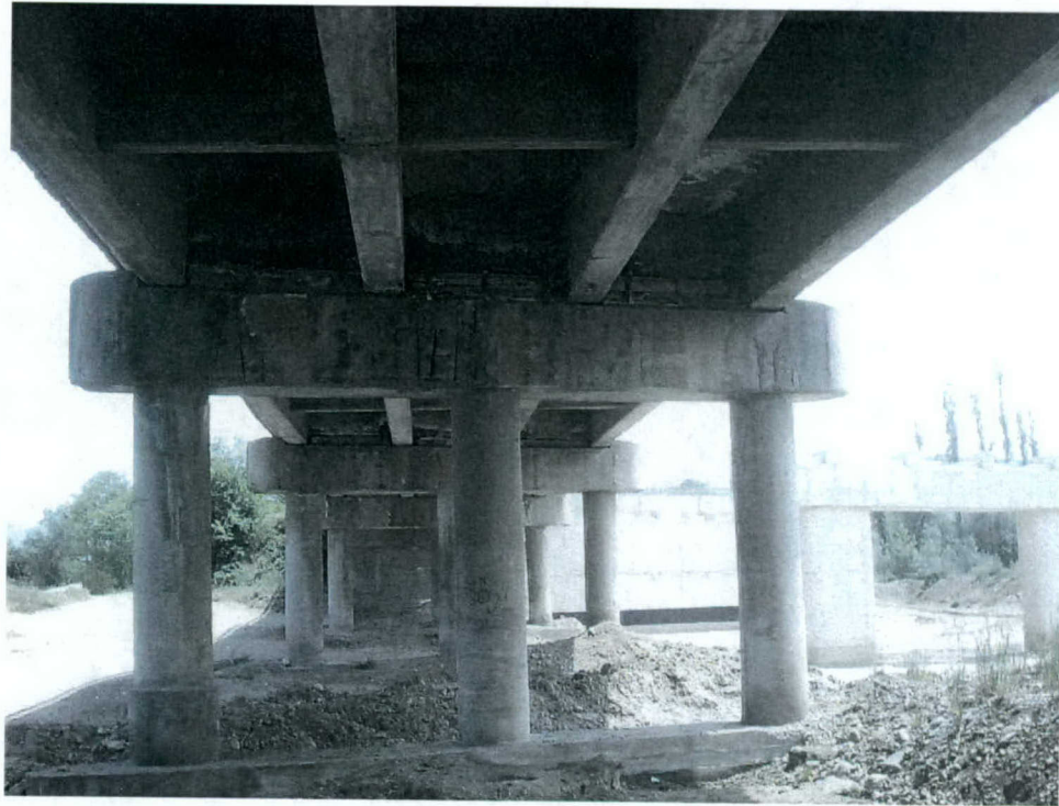
Figure E5. The deck and the pier cap of the Candir Bridge
