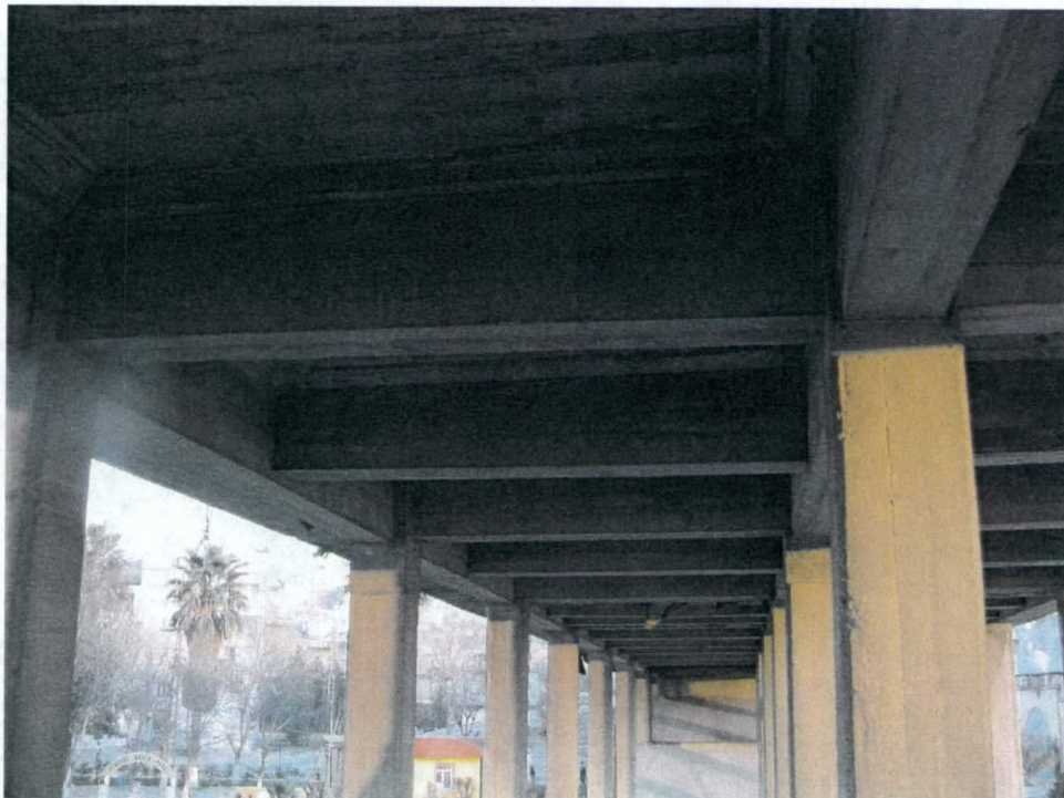
Figure D8. A detail of column-beam-diaphragm connection of the Birecik Bridge
