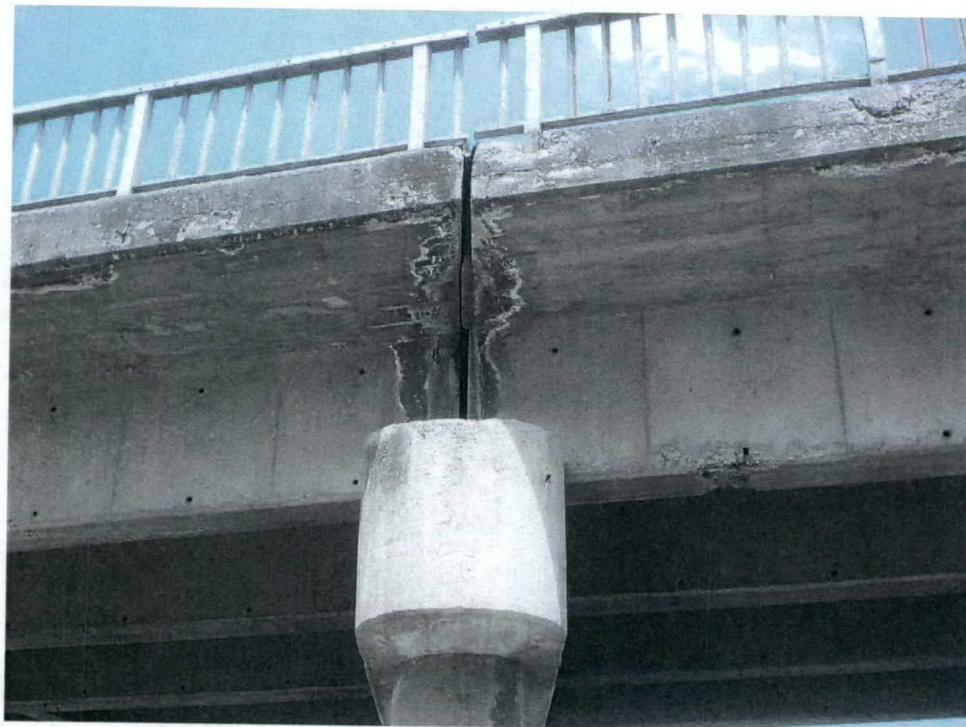
Figure E8. The simple span support of the Candir Bridge
