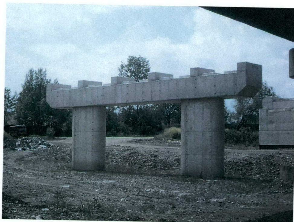
Figure E12. The pier of the new bridge
