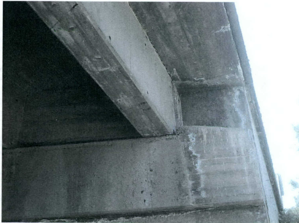
Figure E10. The girder of the Candir Bridge resting on an abutment
