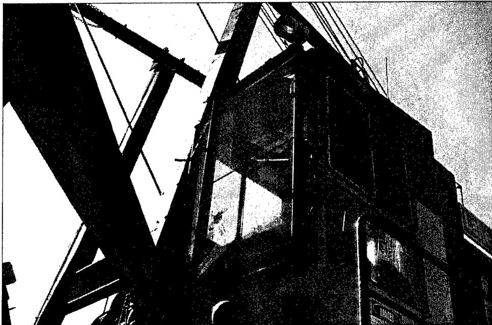
Figure 7. Crane operator's protective barrier
