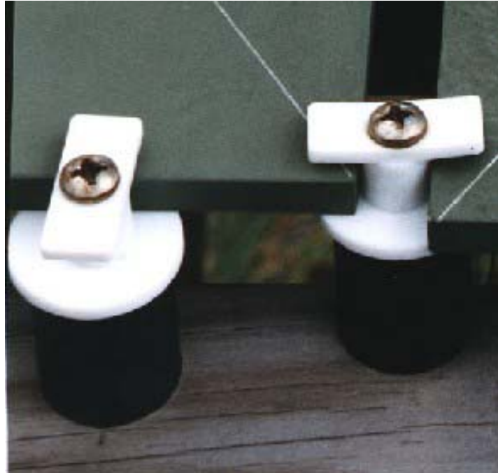
Figure 2. Teflon hold-down brackets.
