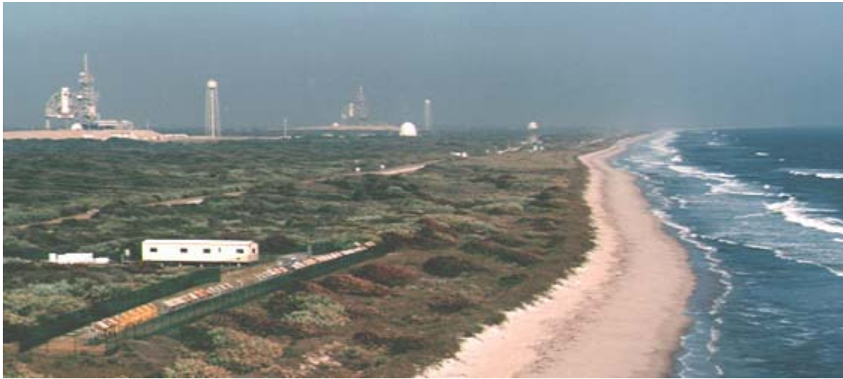
FIGURE 3. View of Beach Corrosion Site and coupon configuration
