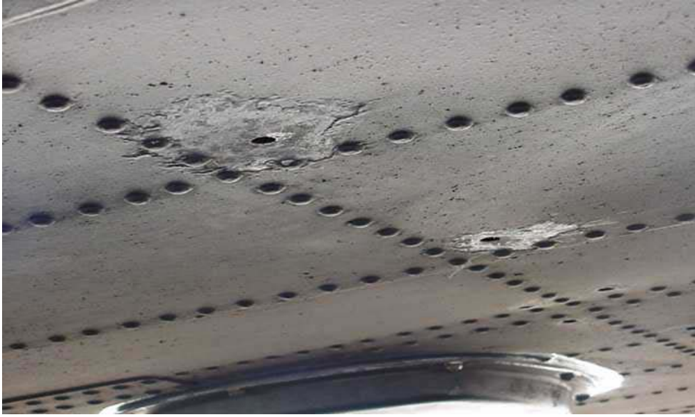
FIGURE 7. External Filiform Corrosion on UH-60 Skin
