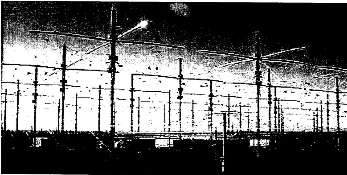
*Figure 4. View of the present 960 kW, 48 element, HF antenna array at Gakona. The planned full array will have 180 elements, and will radiate 3.6 MW.*
