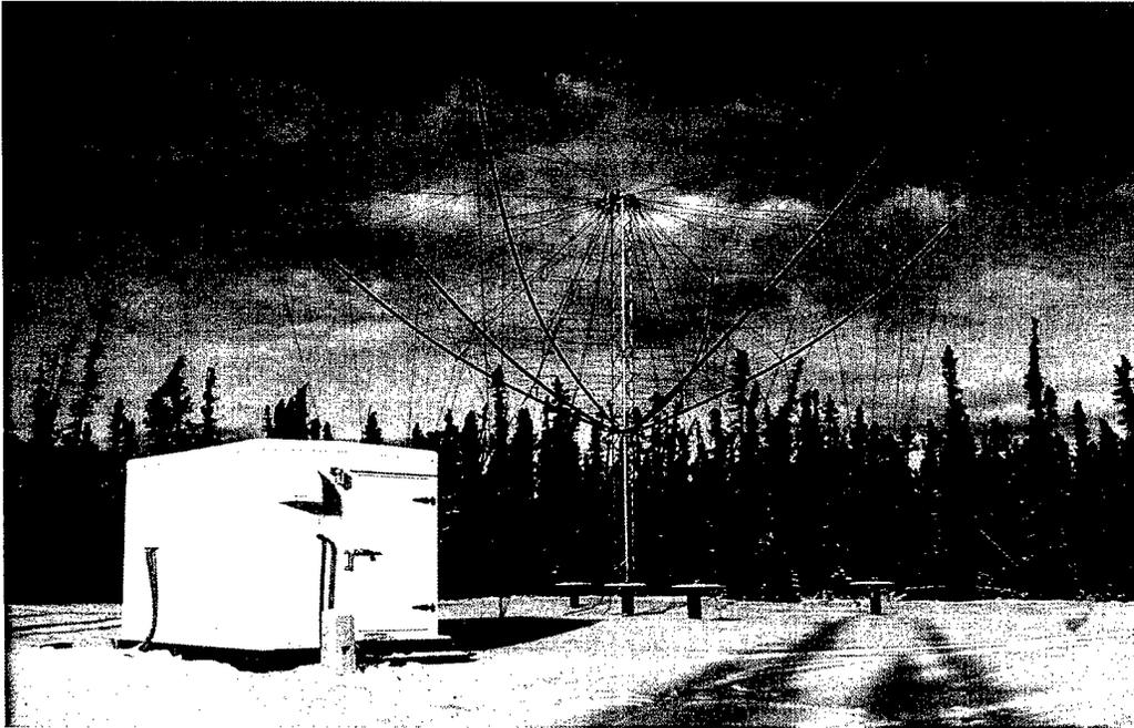
*Figure 12. Pad 2 with HF Spiracone receiving antenna.*
