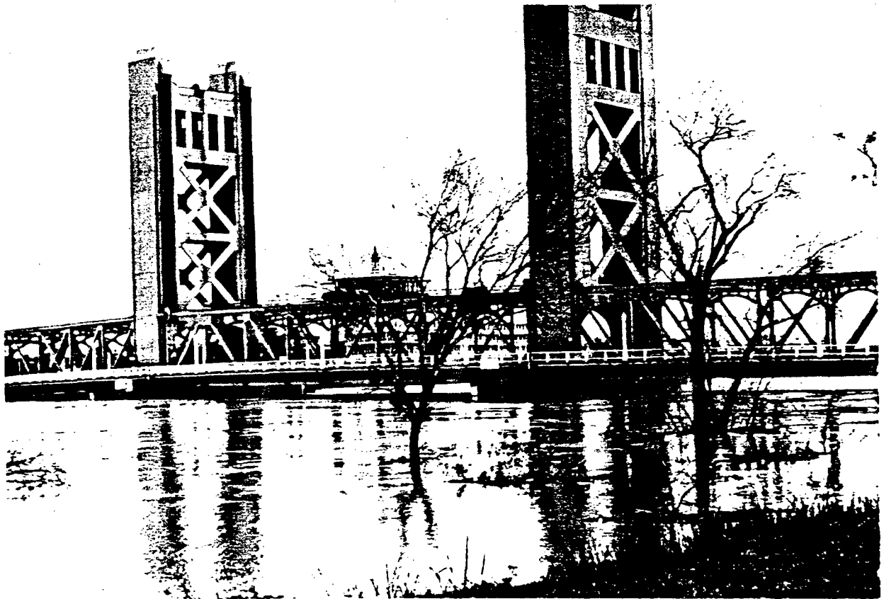
SACRAMENTO RIVER AT TOWER BRIDGE DURING FEBRUARY 1986 FLOOD.
