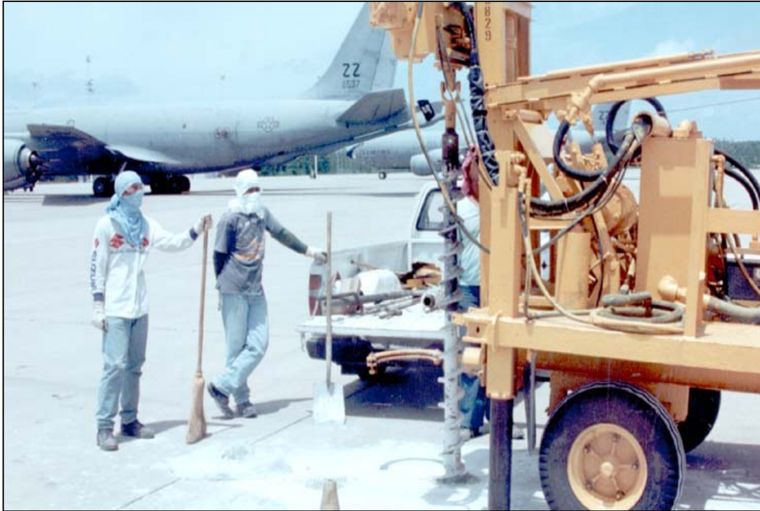
Drilling Bioslurper well on Ramp
