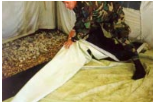
Figure 32. Flooring Section Installation.
