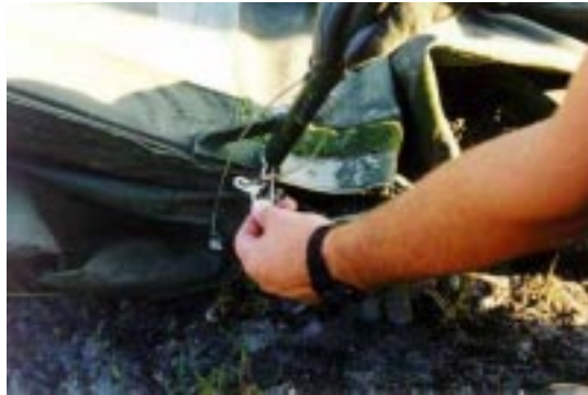
Figure 23. Installation of Eave Extenders.
