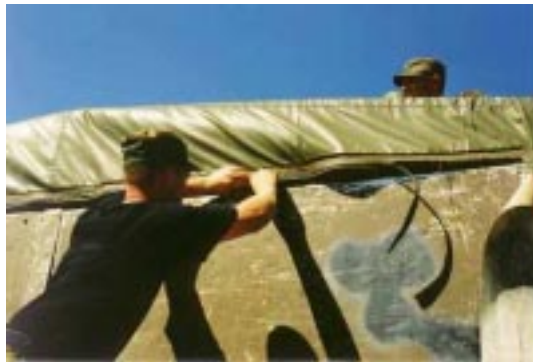
Figure 83. Attaching End Wall Flashing to End Wall Panels.
