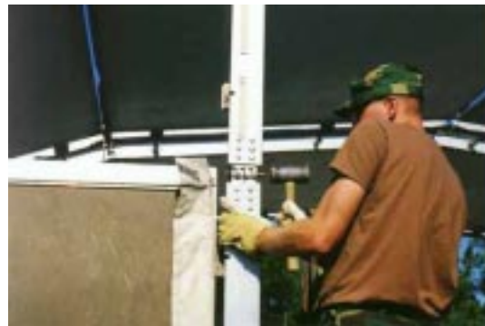
Figure 78. L2/LU-2 Column Connection.
