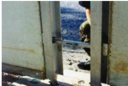
Figure 71. Spacer Bar Attachment.
