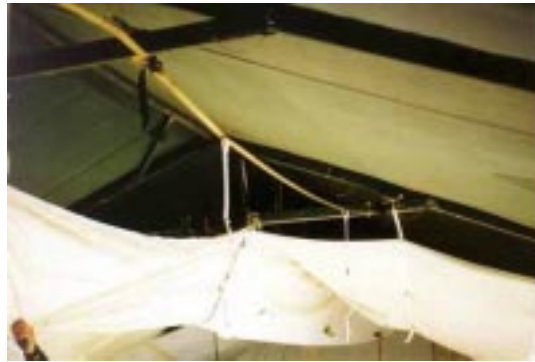
Figure 34. Light Support Strap Assemblies.
