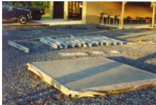
Figure 54. Basepads, Beams and Panels.
