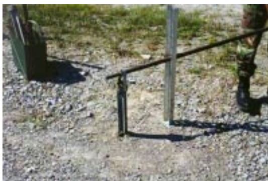
Figure 86. Pulling Shear Stakes.
