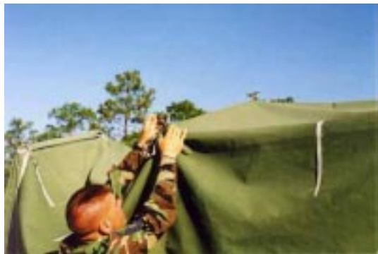
Figure 40. Vestibule Frame Installation.
