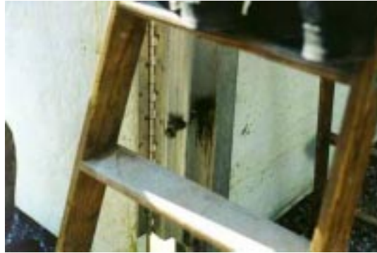
Figure 81. Door Hinge Mounting Bolts and Column Mounting Inserts.
