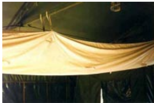
Figure 5. Fabric Plenums.
