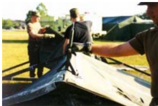
Figure 20. Installation of Ridge Extenders.
