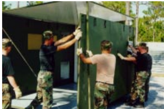
Figure 47. Raising of End Wall.
