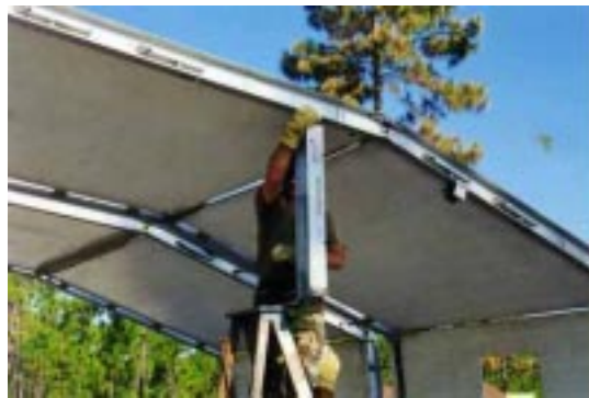
Figure 77. Installation of Header.
