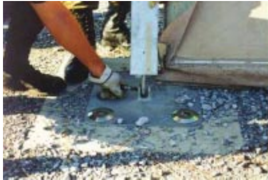
Figure 63. Pinning of Panel to Basepads.
