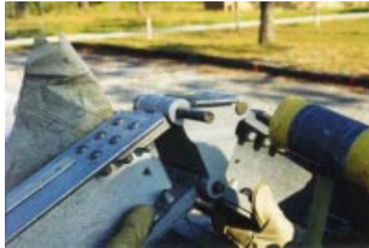
Figure 62. Beam-to-Beam Pin Connection.
