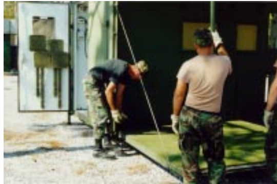
Figure 46. Safety Cable Attachment.
