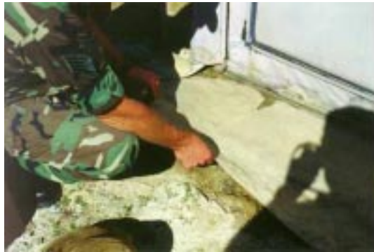
Figure 85. Installation of Ground Skirt Flashing.
