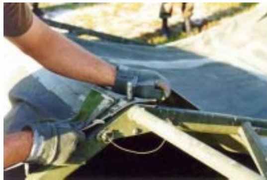
Figure 16. Large Grommet Placed Over Ridge Joint Spindle.
