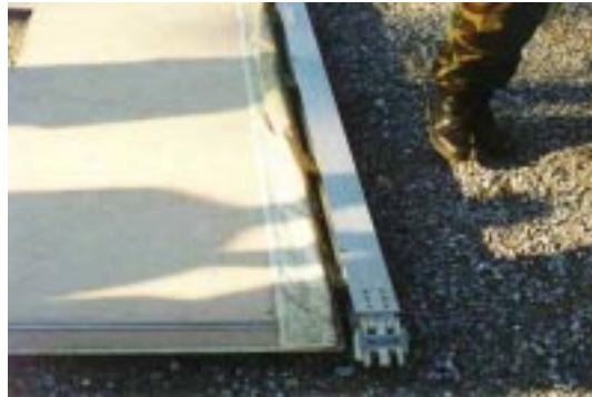
Figure 61. Panel-to-Arch Beam Connection.
