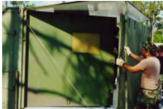
Figure 48. Positioning of Swing-out SideWalls.
