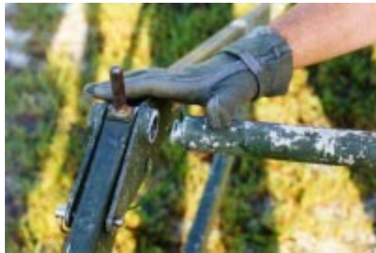
Figure 11. Purlin-to-Arch Connection.
