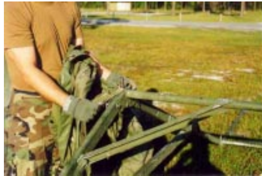
Figure 20. Installation of Ridge Extenders.
