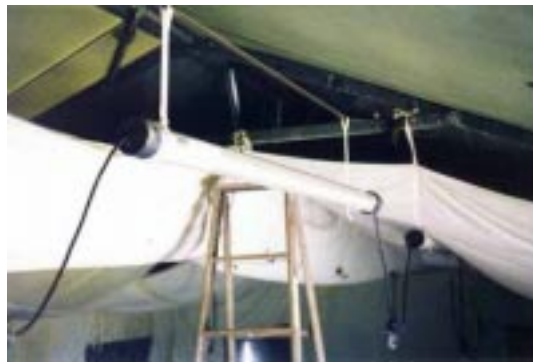
Figure 38. Installation of Light Fixtures.
