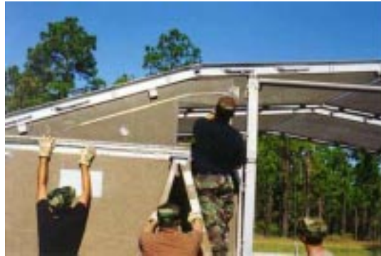
Figure 79. Upper Panel Section Placement.
