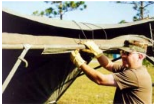
Figure 29. Securing Purlin Flaps.
