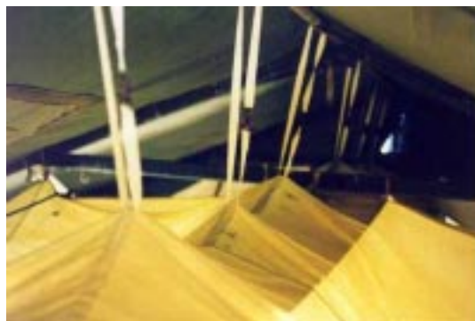
Figure 35. Overhead Liner Connections.
