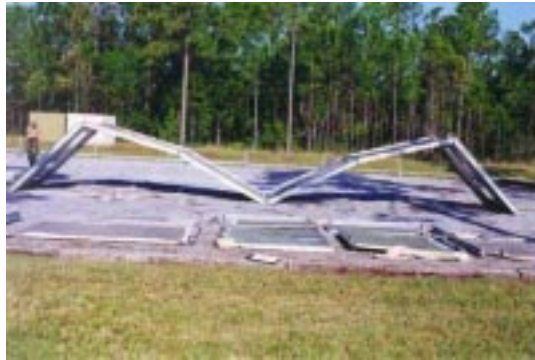
Figure 65. Placement of Panel Sections Prior to Erection.
