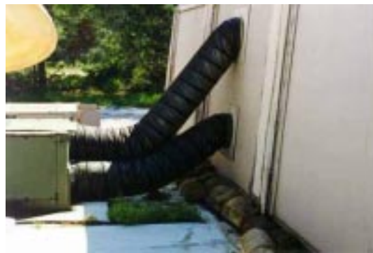
Figure 70. Bare Base Environmental Control Unit Attached to GP Shelter.
