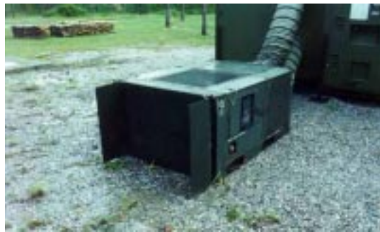
Figure 51. Environmental Control Unit Installation.
