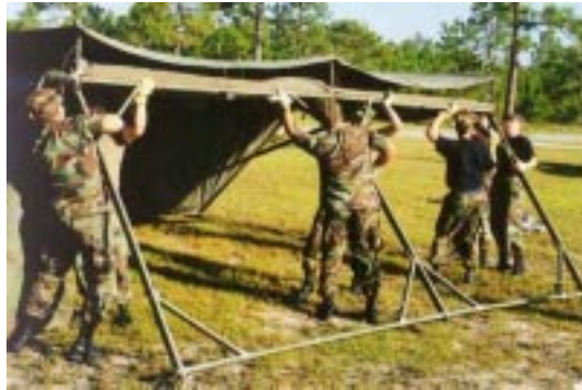
Figure 27. Raising of Tent Frame Assembly.
