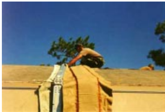
Figure 84. Arch Counterflashing Attachment.
