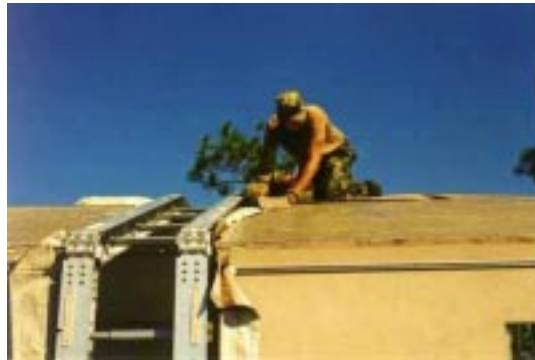
Figure 75. Ridge Flashing Installation.
