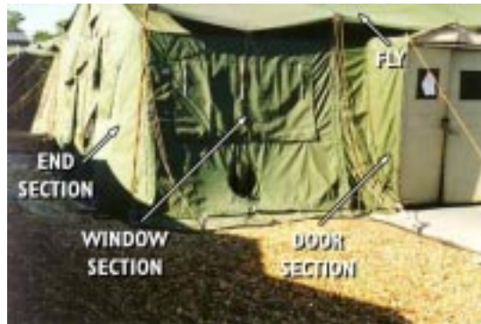
Figure 2. TEMPER Tent Fabric Components.
