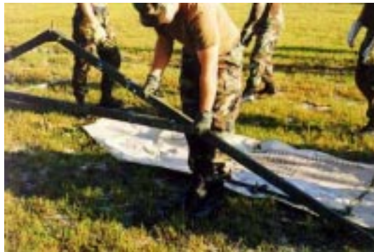
Figure 10. Header Assembly.
