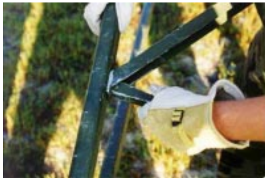
Figure 13. Rotation of Tab Handle to Lock Tab Into Arch.
