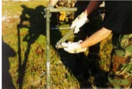
Figure 13. Rotation of Tab Handle to Lock Tab Into Arch.
