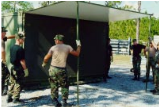
Figure 45. Raising of Roof Panel.
