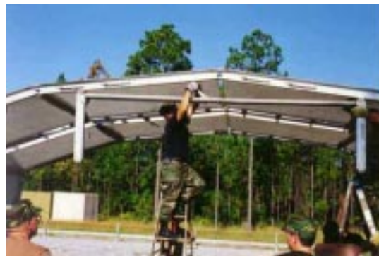
Figure 77. Installation of Header.
