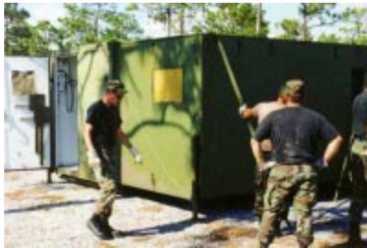
Figure 49. Final Positioning of Expanded Section.
