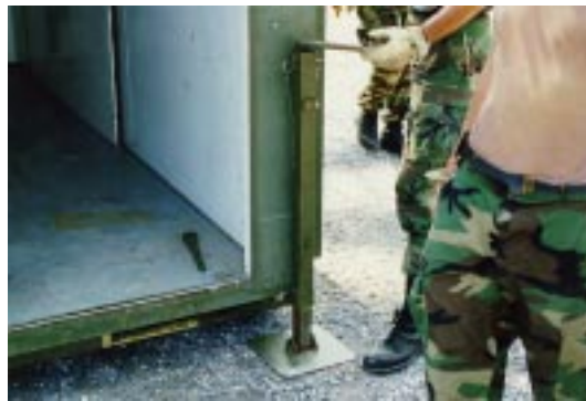
Figure 44. Leveling Center Section.
