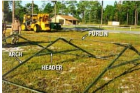
Figure 3. TEMPER Tent Frame Components.
