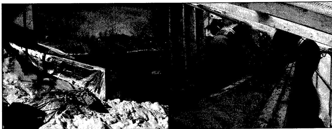
Figure 81. NHDOT crew placing regular concrete (left) within the confines of a heated tent (right) during bridge curb repairs in West Lebanon. This pour, on the east side of the Trues Brook bridge, was the mirror opposite of the antifreeze concrete repair performed on the west side.
