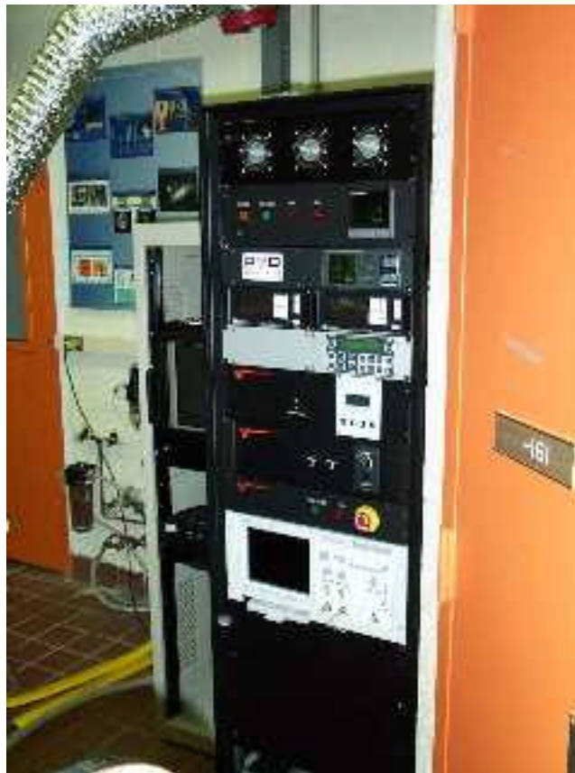
Figure 44 Main Control Rack
