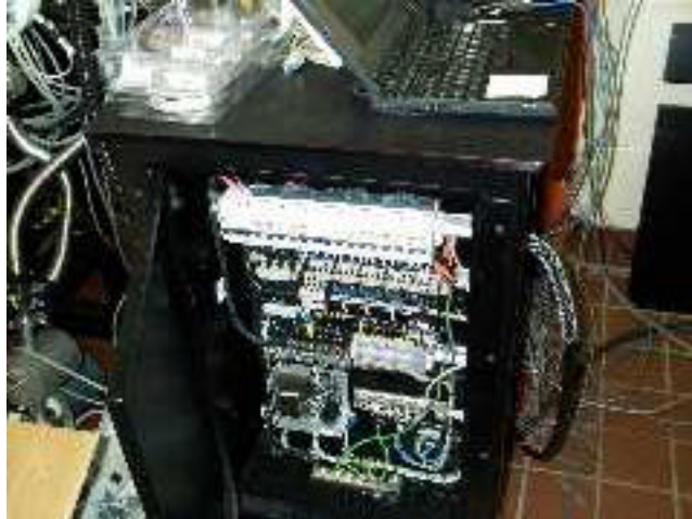
Figure 46 Power Distribution Rack
