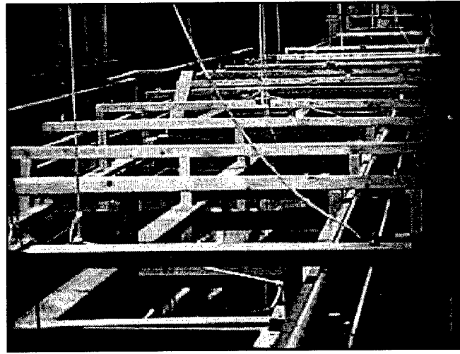
Figure 14. Ice restraint system upstream.
