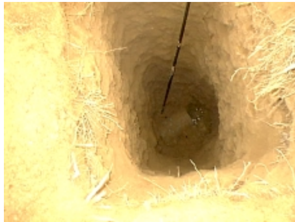
Typical excavation at JPG IV
