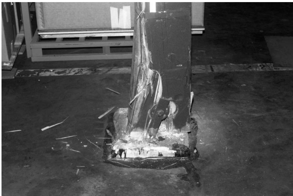
Figure 11. Retro-reflective tape marker (top, center) on displaced support column after being struck by fork truck.
