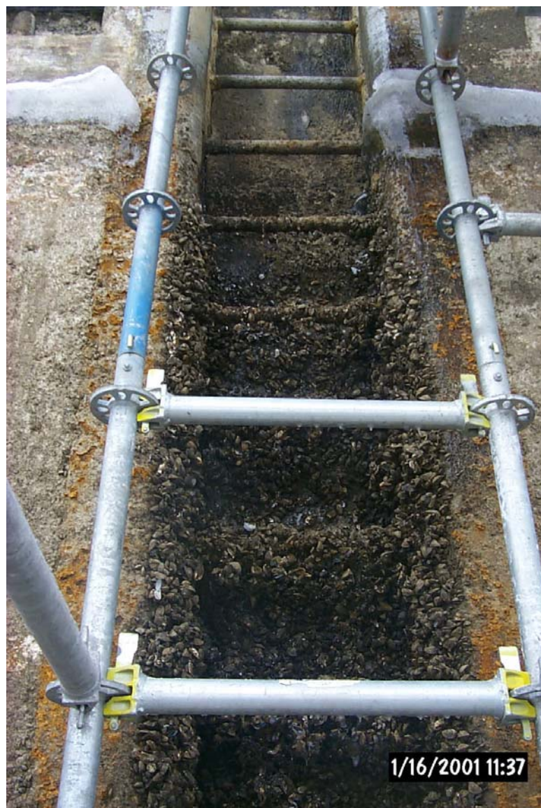
b. Recessed ladder well.
