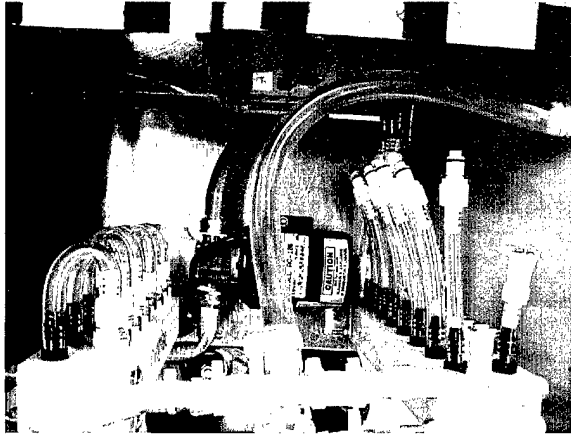
(a) Top view of the water coolant distribution manifold. The water circulation pump is visible at the back of the picture (bottom of the rack). A few circuit boards (one per channel) are visible mounted in the rack.
