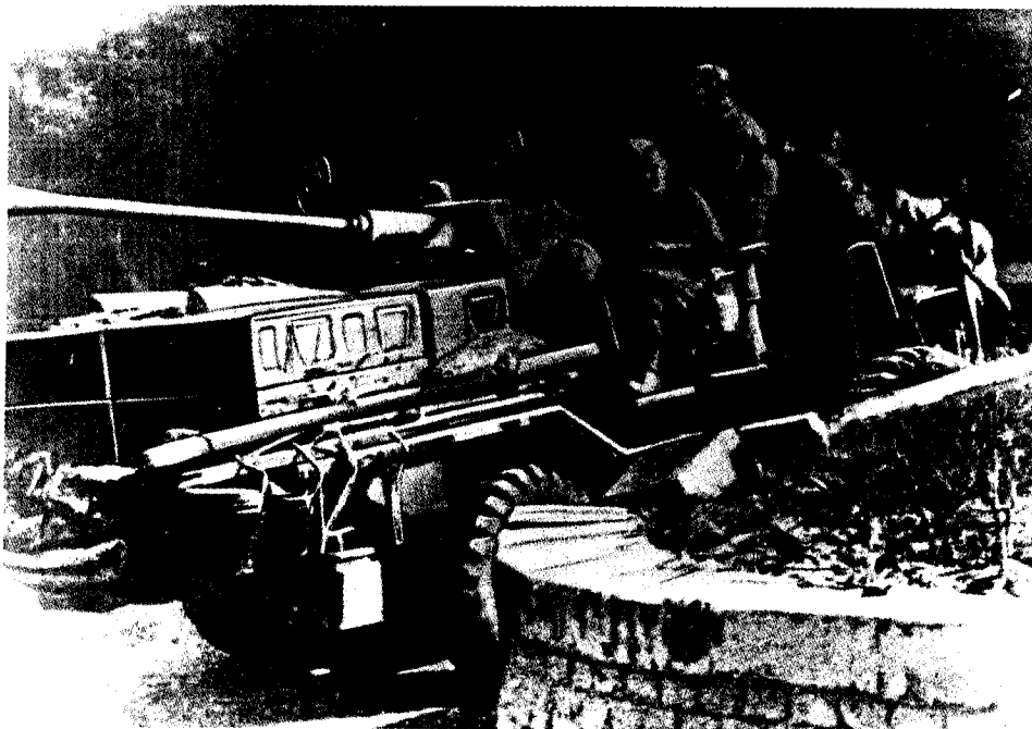
Figure 23. German light flak pieces were also mounted on motor vehicles. Here a 20-mm gun is seen with a makeshift mount on an Opel truck.
