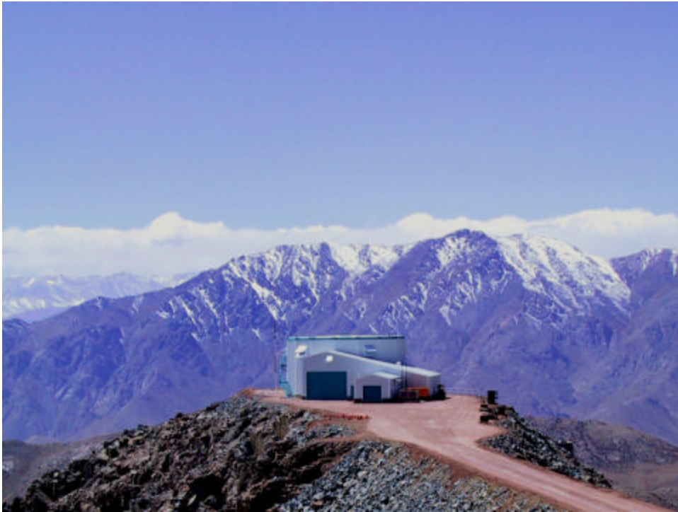
Figure 2. The SOAR facility on Cerro Pachon in northern Chile prior to installation of the dome in March 2002
