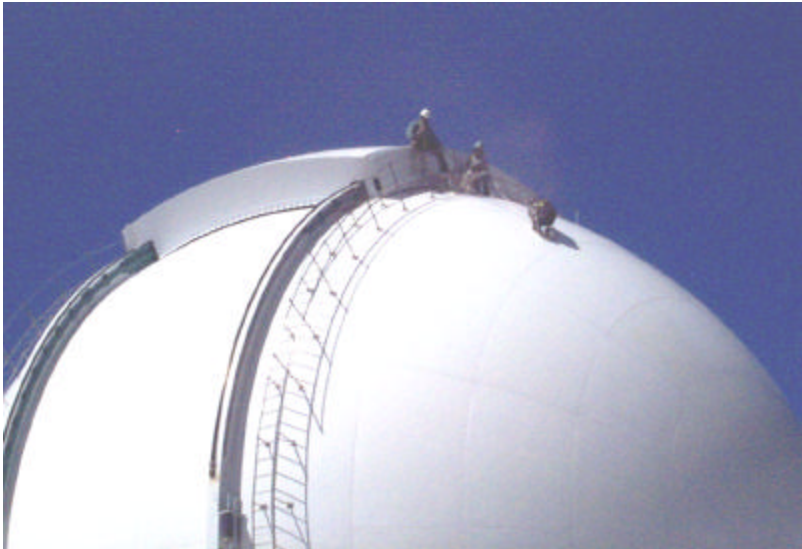
Figure 5. Exterior of the SOAR dome being painted.
