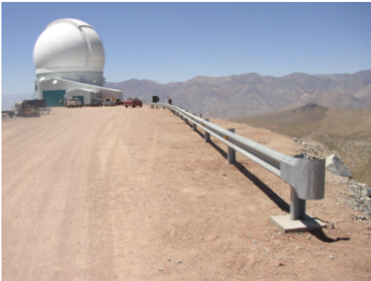
Figure 3. The SOAR site. View of SOAR from access road; installation of guardrail.
