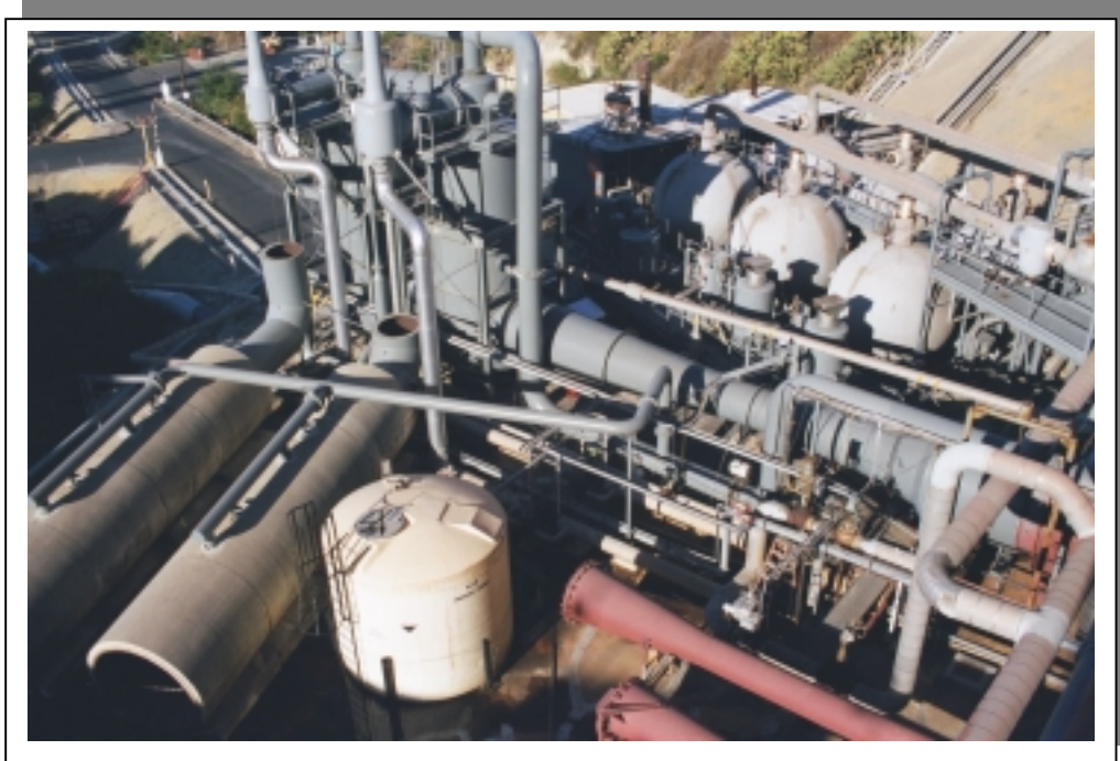
Steam plant and cooling water at VETS.
