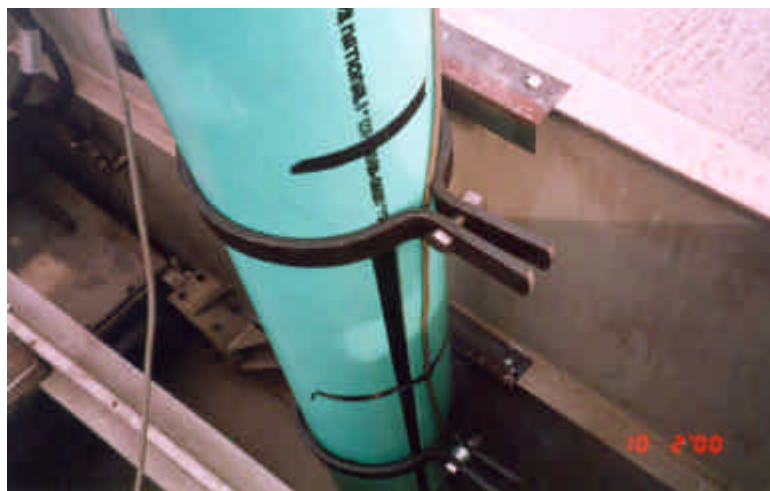
Figure 35. PVC Tube in HSS Collection Well.
