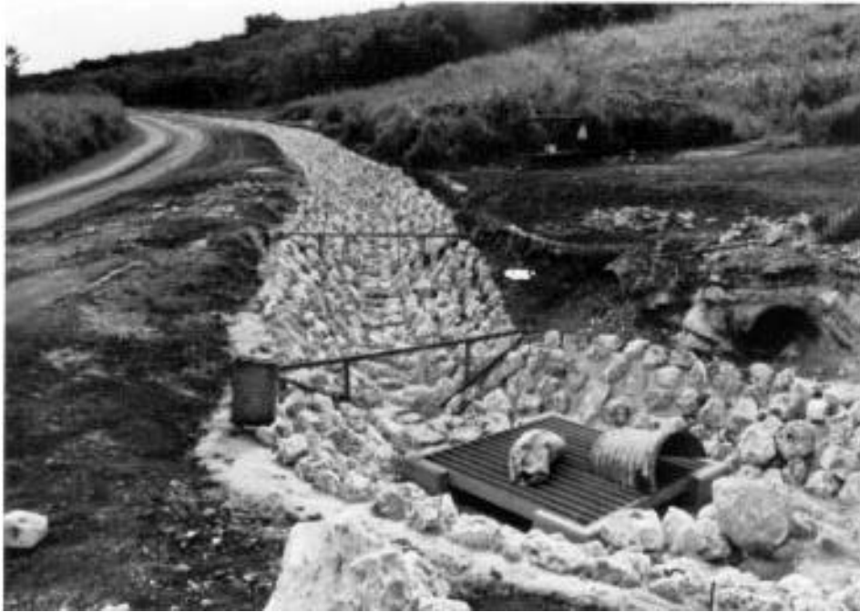
D.14 Looking Northeast into Inlet to Culvert III (work in progress at time of photo)
