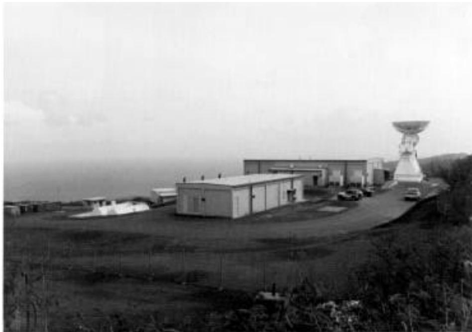
D.29 Looking Northwest toward Radar Site Post-construction
