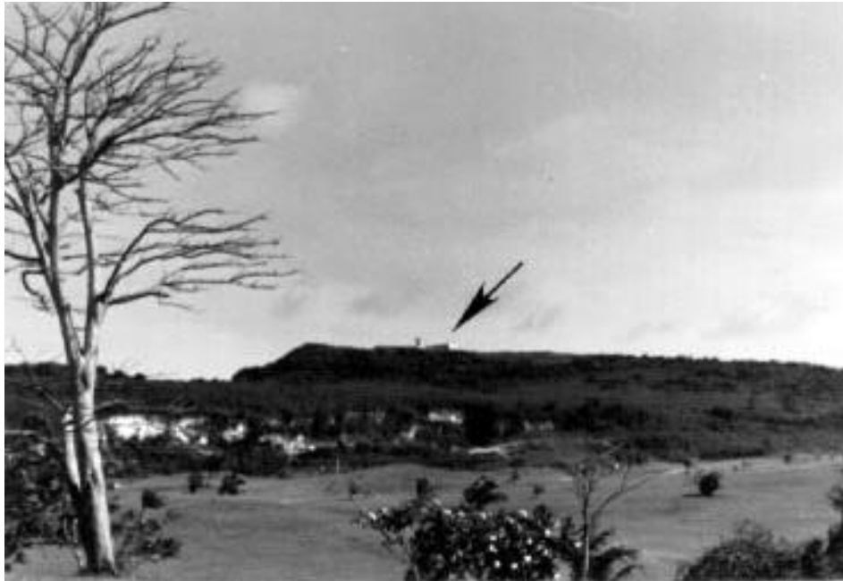
D.4 Looking Southeast from Golf Course Radar Facility atop Hill at Center of Photo
