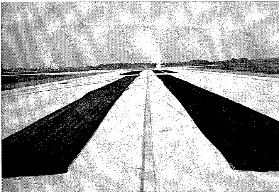
Figure 9. View of Taxiway M after application of test materials but prior to application of CPR material (Figure 7)
