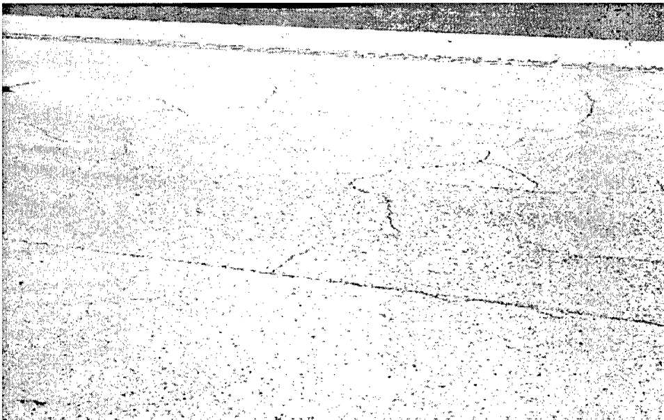
Figure 4. Typical block and longitudinal cracking on Taxiways O and M at MacDill AFB
