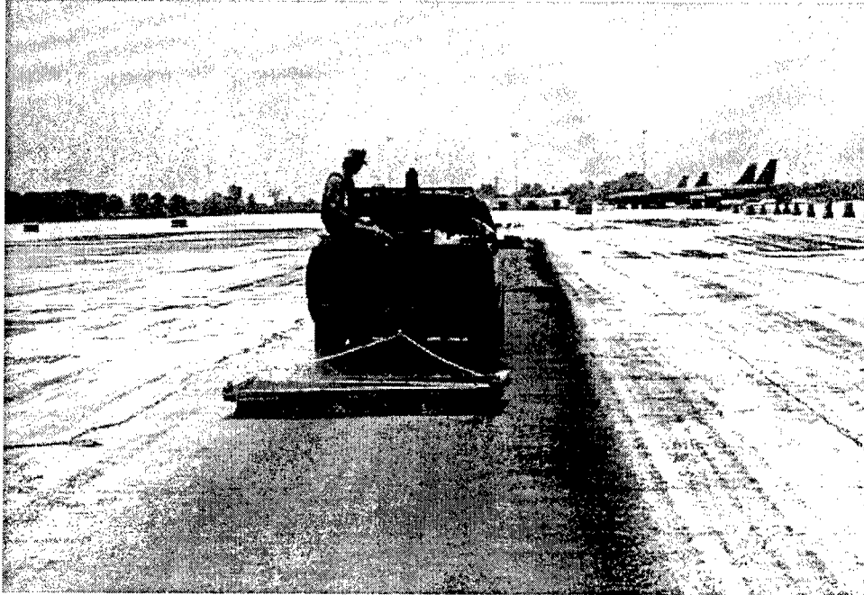
Figure 22. Working sand into the CRF emulsion with a drag broom
