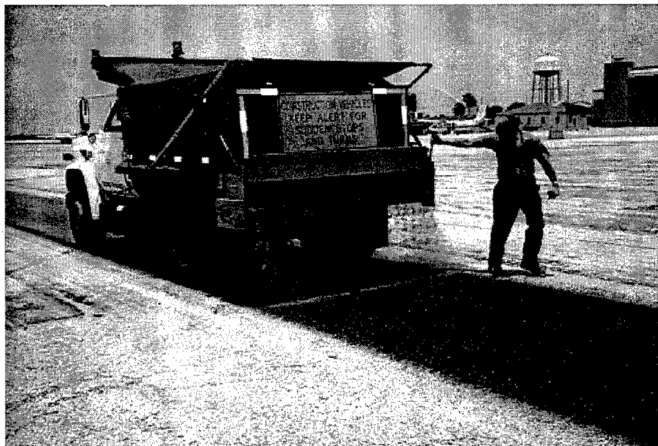
Figure 21. Spreading sand over CRF emulsion
