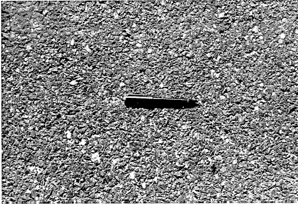
Figure 16. Closeup view of HMA surface on Taxiway L at McGuire AFB
