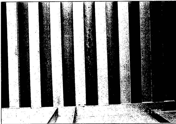
Photo. 25: Moderate corrosion on downstream surface of skin plate.
