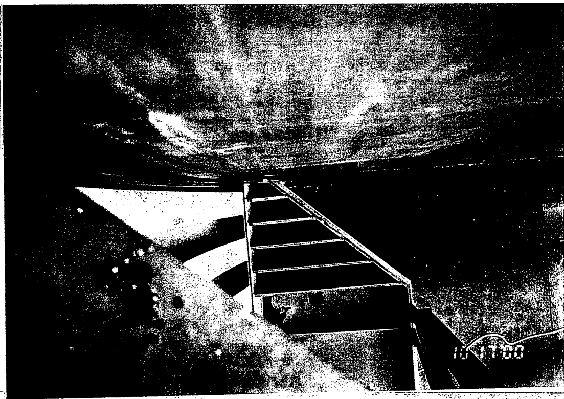
Little Goose Dam 10/17/00 2-5 Gate 2 Bottom horizontal girder, left end. Standing water, no drainage between multiple stiffeners, typical.
