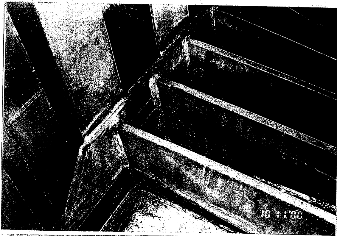
Little Goose Dam Gate 7 Bottom horizontal girder, left end. Standing water, no drainage between multiple stiffeners, typical. 10/11/00 7-12
