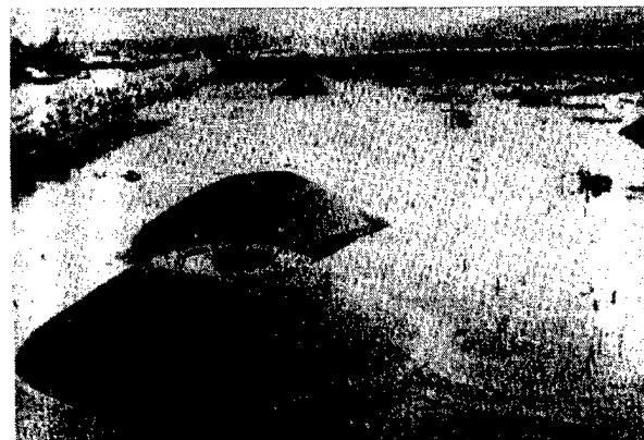
Figure 3-13. Sand boils at Friars Point, Mississippi
