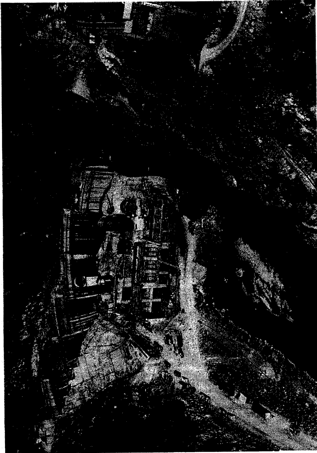
Figure 13-6. Channel used in the Phase I diversion for Smith Mountain Dam (photograph courtesy of Appalachian Power Company)
