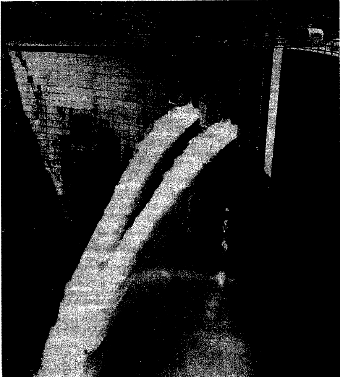
Figure 3-2. Through spillway below crest on Morrow Point Dam (USBR)
