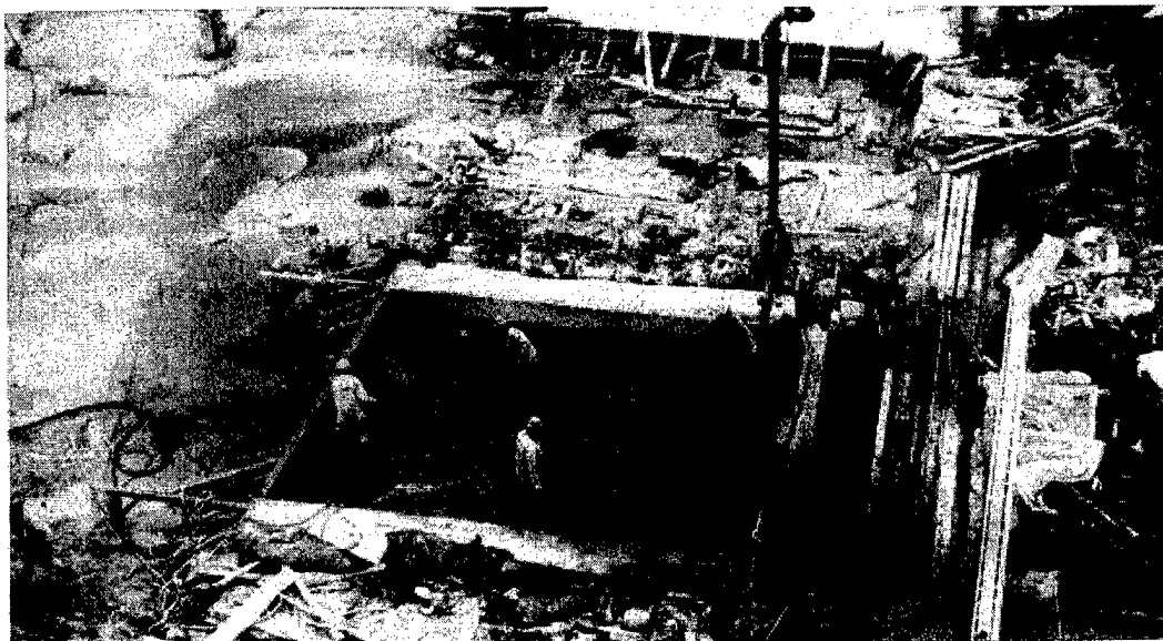
Figure 8-36. Pumping silica-fume concrete into the stilling basin from the top of the right training wall, Kinzua Dam
