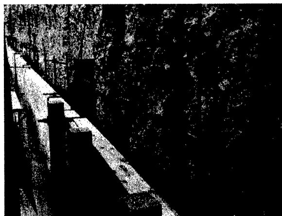
Figure 8-15. Installation of precast concrete stay-in-place forms at Troy Lock, Hudson River (Miles 1993)
