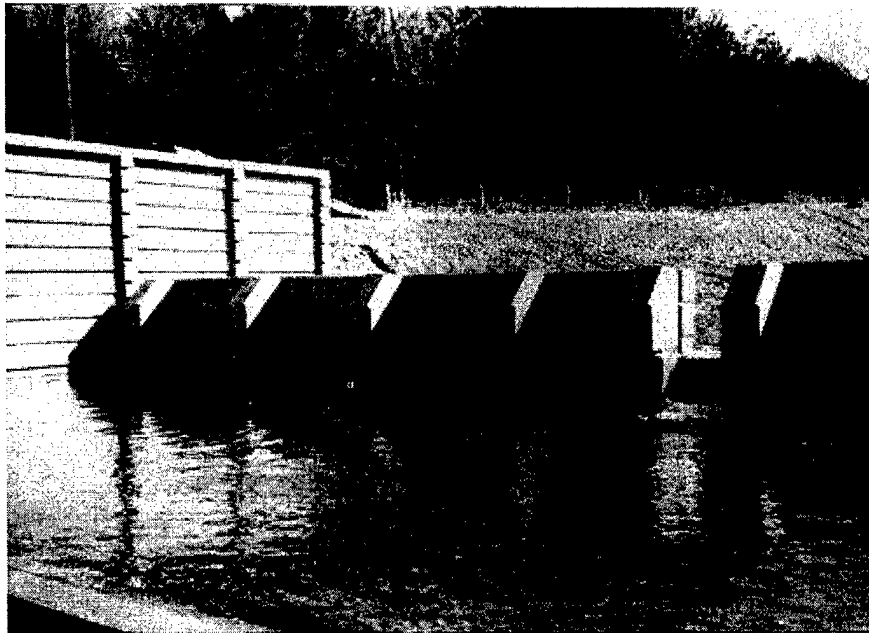
Figure 8-43. Precast concrete checkdams, Chauncy Run
