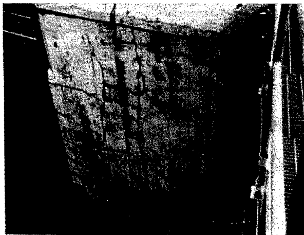
Figure 8-16. Typical cracking in miter gate monoliths resurfaced with cast-in-place concrete, Troy Lock, Hudson River (Miles 1993)
