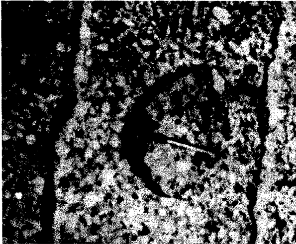
Figure 2-29. Small spall
