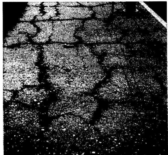
Figure 2-6. Pattern cracking resulting from alkali-silica reaction
