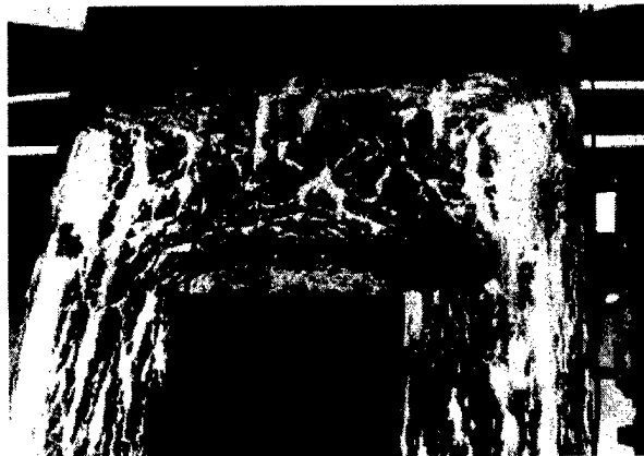
Figure 2-24. Efflorescence
