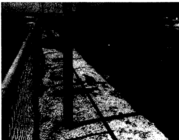
Figure 2-18. Severe scaling
