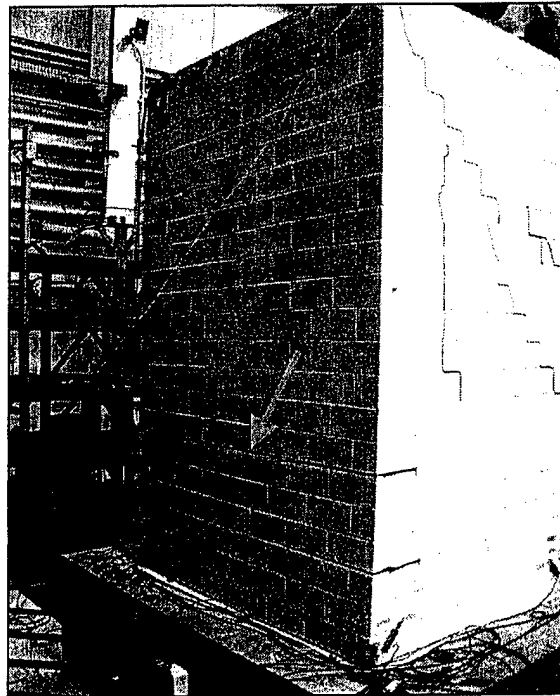
Figure 7.9. Actual bed-joint cracking characteristic of pier rocking (Test 11, Specimen #1).
