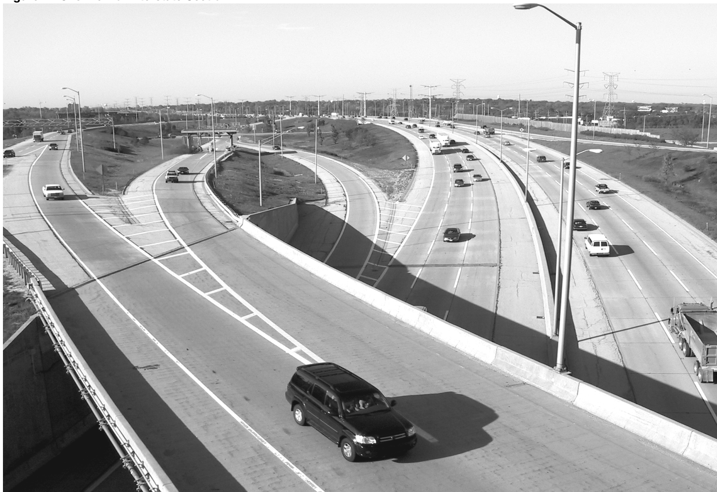
Figure 2: Overview of Interstate Section
