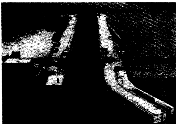
Figure 2-2. Lock with gravity walls. Lower Granite Locks, Snake River, with design lift = 100 ft
