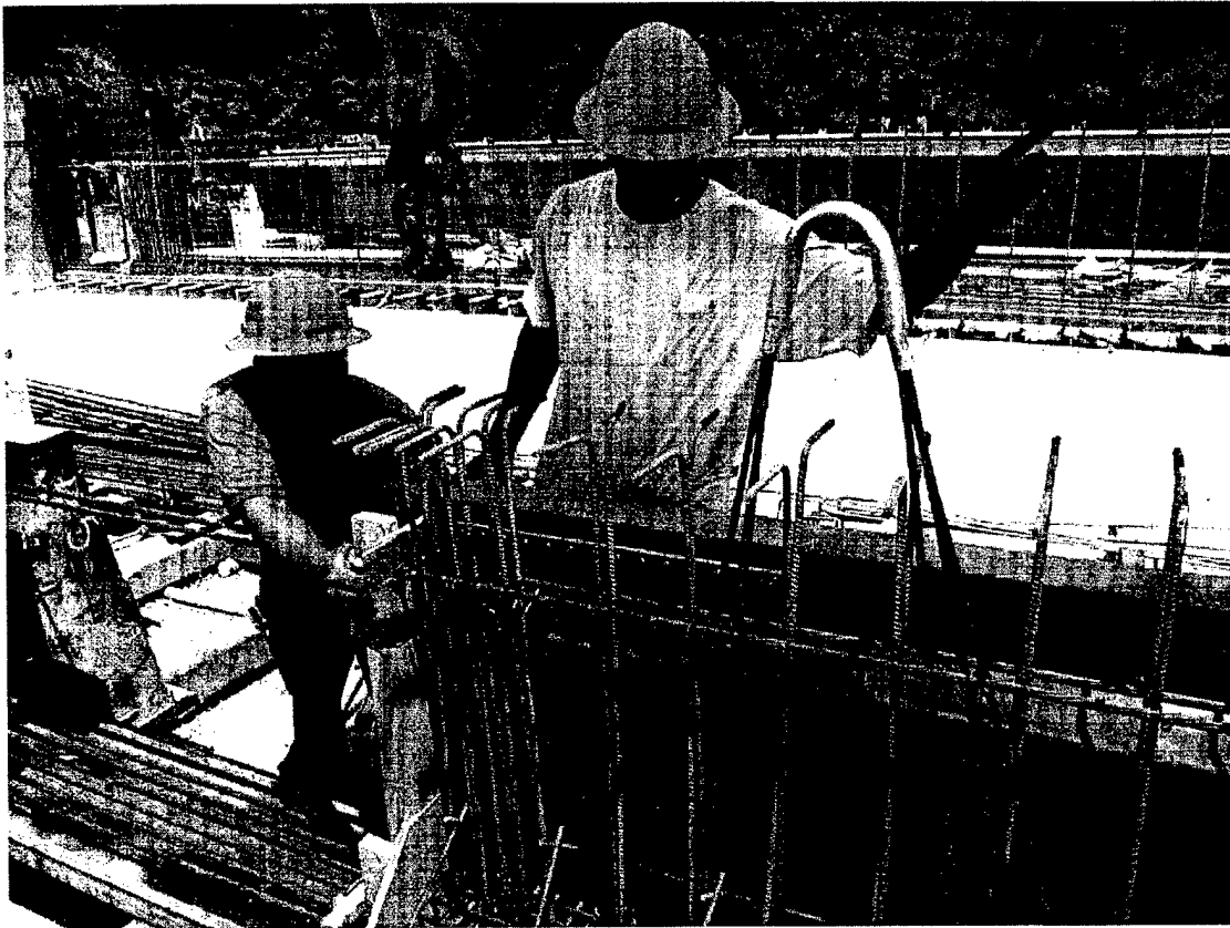
Figure 8.29 Tindall Supervisor Directing Placement of Formwork.
