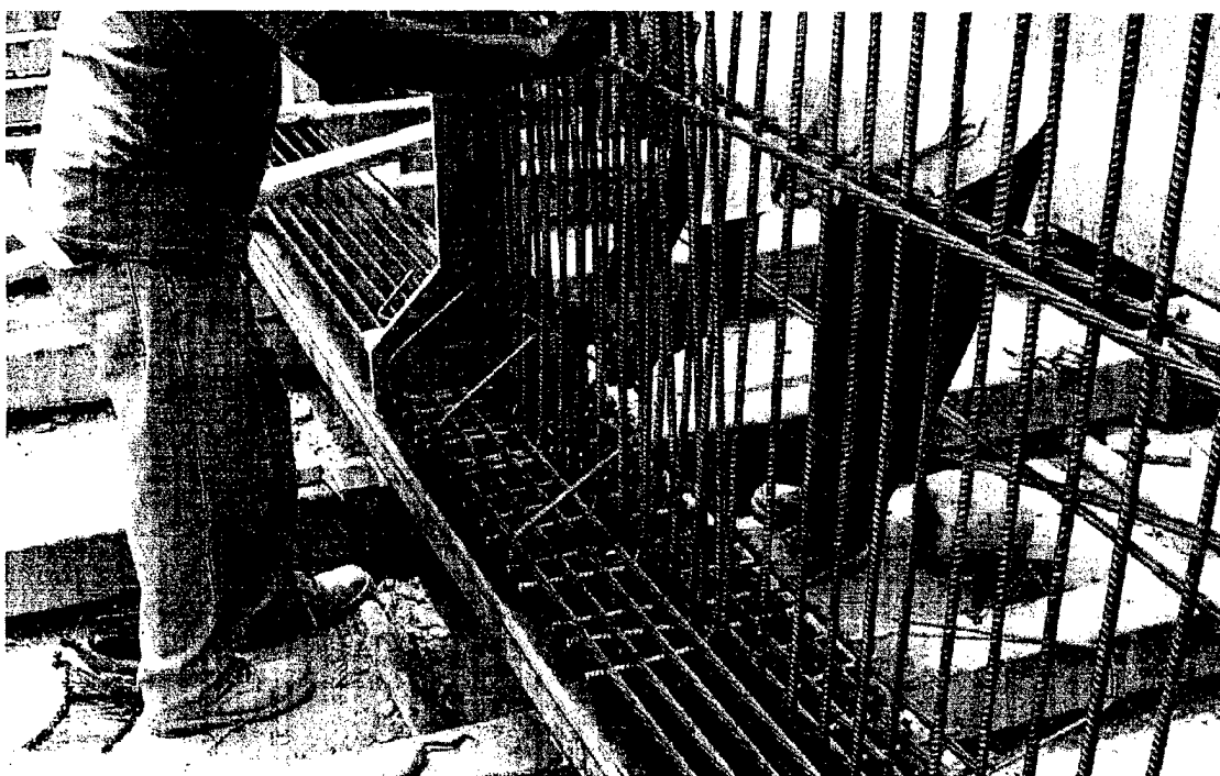
Figure 8.27 Installation of Shear Reinforcing Steel Near Girder End
