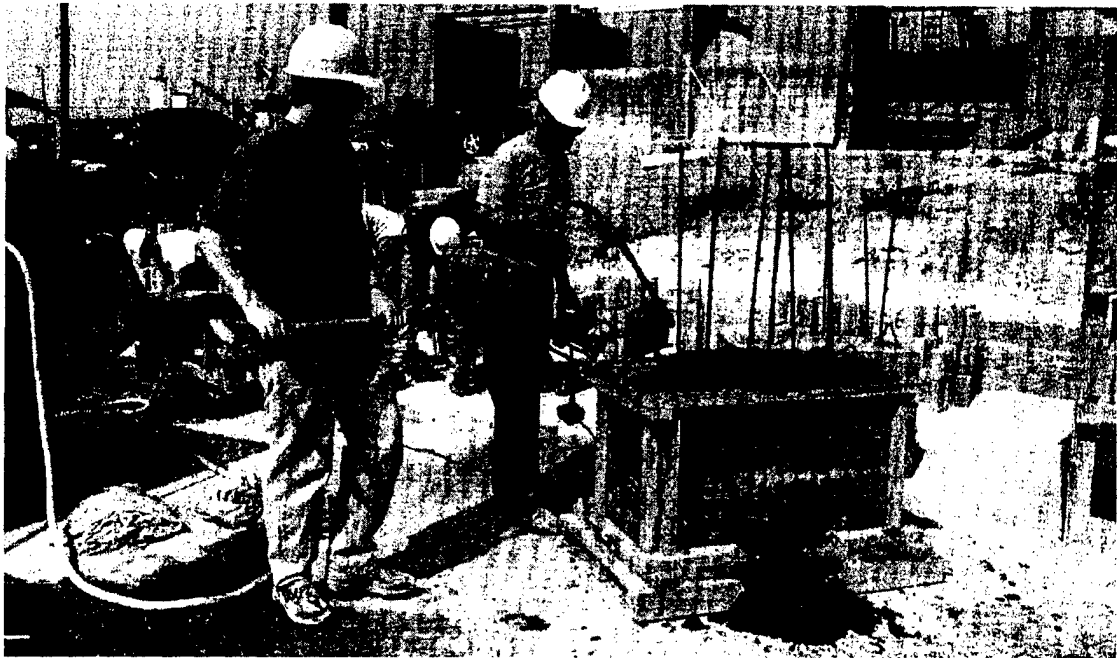
Figure 4.11 Casting of Block for Direct Pullout Test at Tindall Concrete Plant
