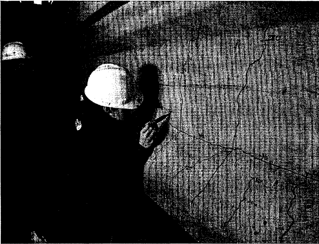
Figure 10.8 Marking of Cracks During Girder Test
