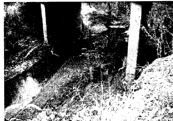
Figure 4-11. Exposed bridge piling
