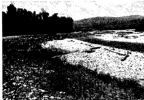
Figure 3-8. Bank protection necessitated by encroachment on levee setback
