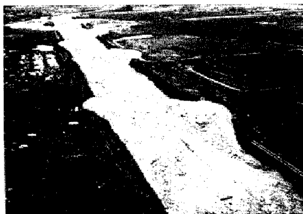
Figure 3-6. Lateral instability in realigned channel
