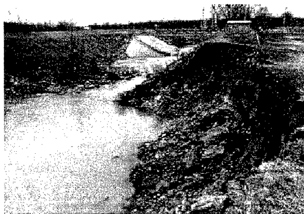
Figure 4-6. Bank failure
