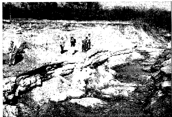
Figure 3-13. Grapevine Spillway Channel after erosional episode
