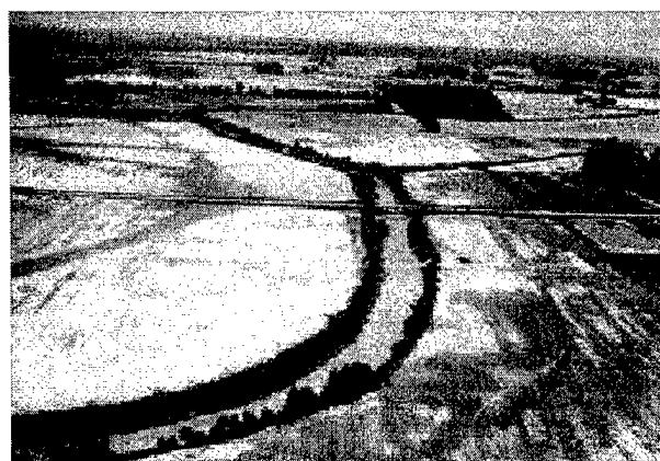
Figure 3-5. Realigned channel without serious instability problems
