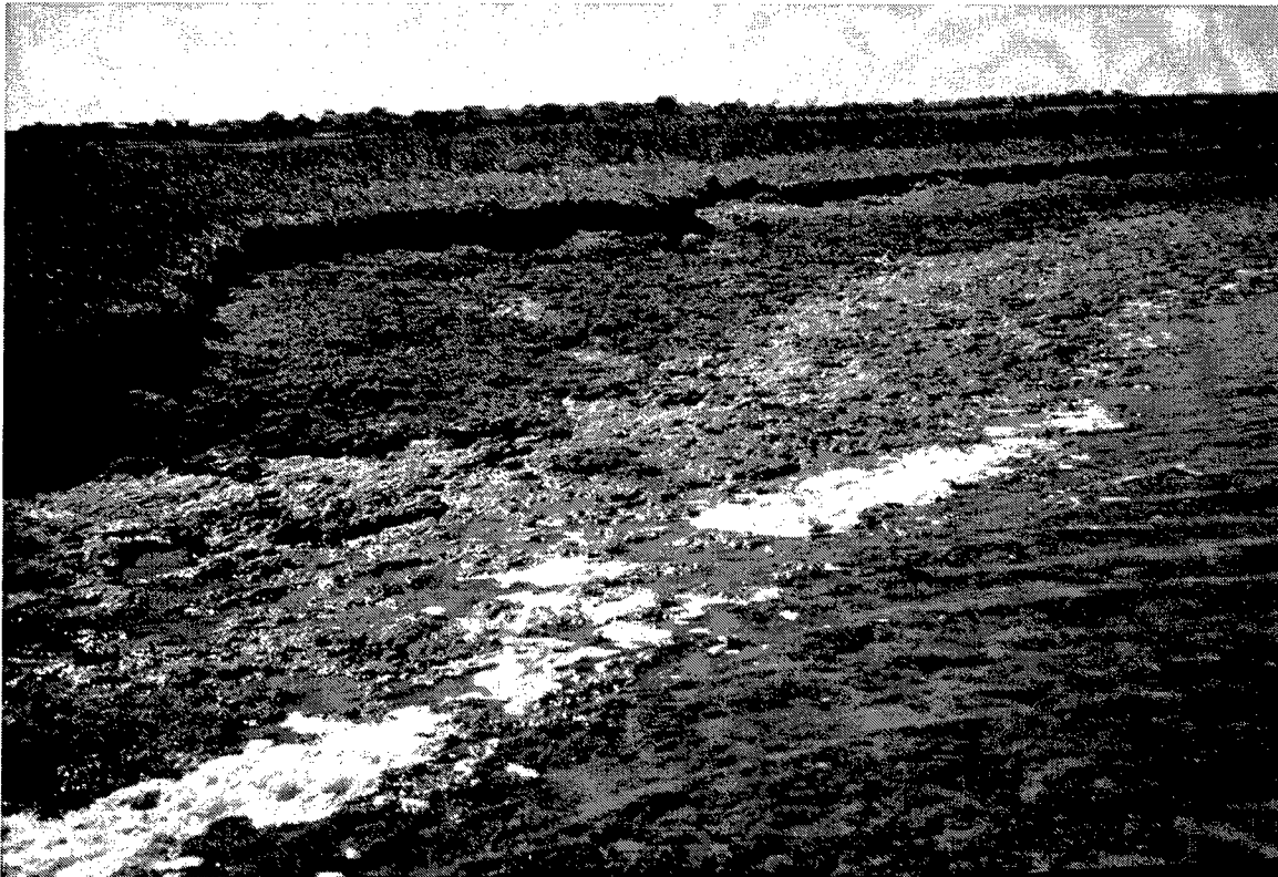
Figure D1. Marsh shoreline exhibiting evidence of erosion (e.g., vertical bank, exposed roots, slumping bank)
