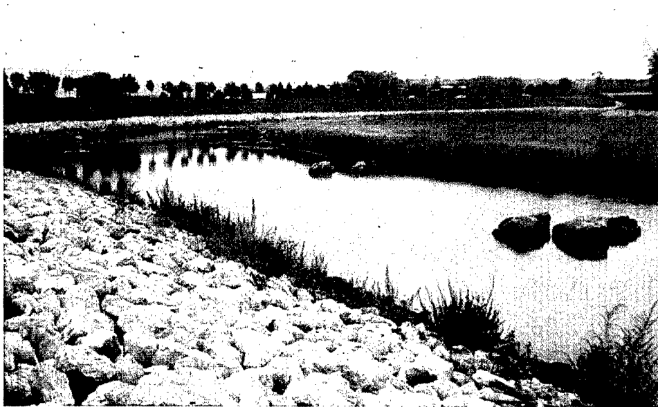
Figure 13. Project designed for flood protection with habitat enhancement features boulder clusters and low-flow deflectors, Zumbro River, Rochester, MN
