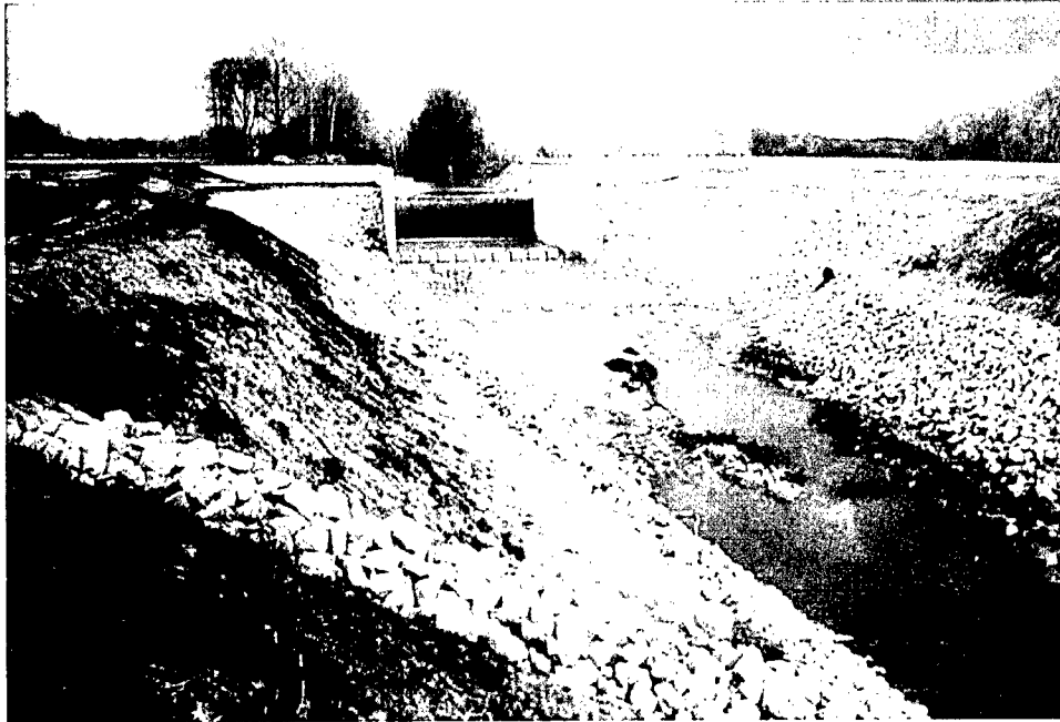
Figure 6. Channel stabilization with grade control, Hotophia Creek, MS
