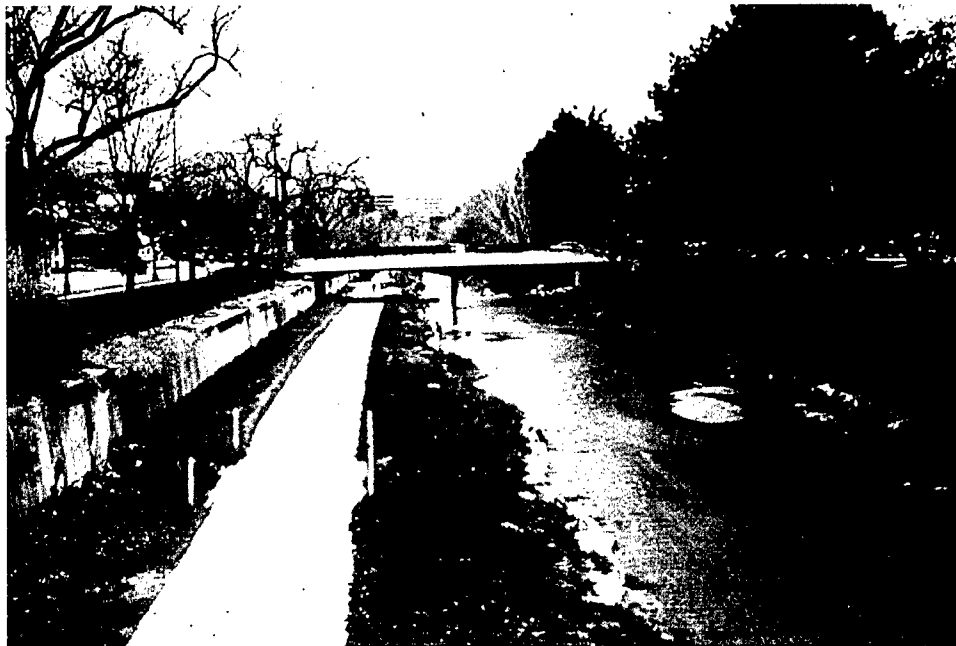
Figure 15. Project designed to provide flood protection, aesthetics, and recreation, Cherry Creek, Denver, CO
