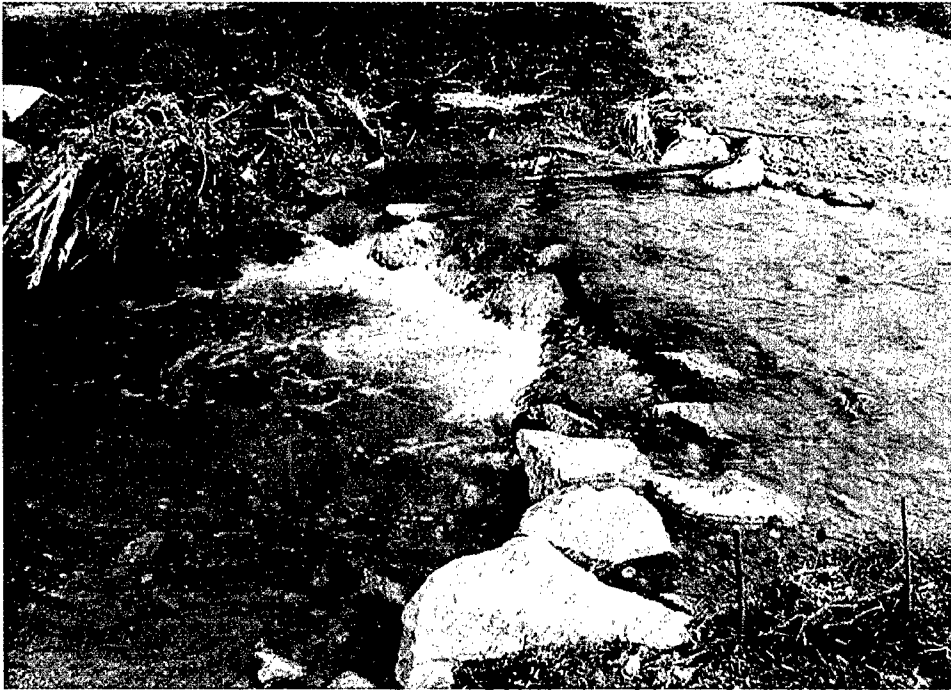
Figure 8. Habitat enhancement with the use of low-flow stone weirs, Paint Branch, MD
