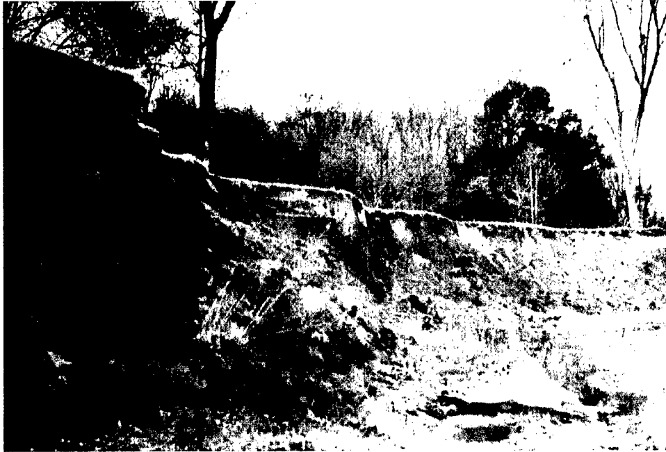
Figure 2. Bank erosion of vegetated bank, Johnson Creek, MS
