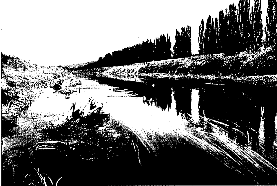
Figure 10. Habitat enhancement features (root wads) added to flood-control project, Sammamish River, WA
