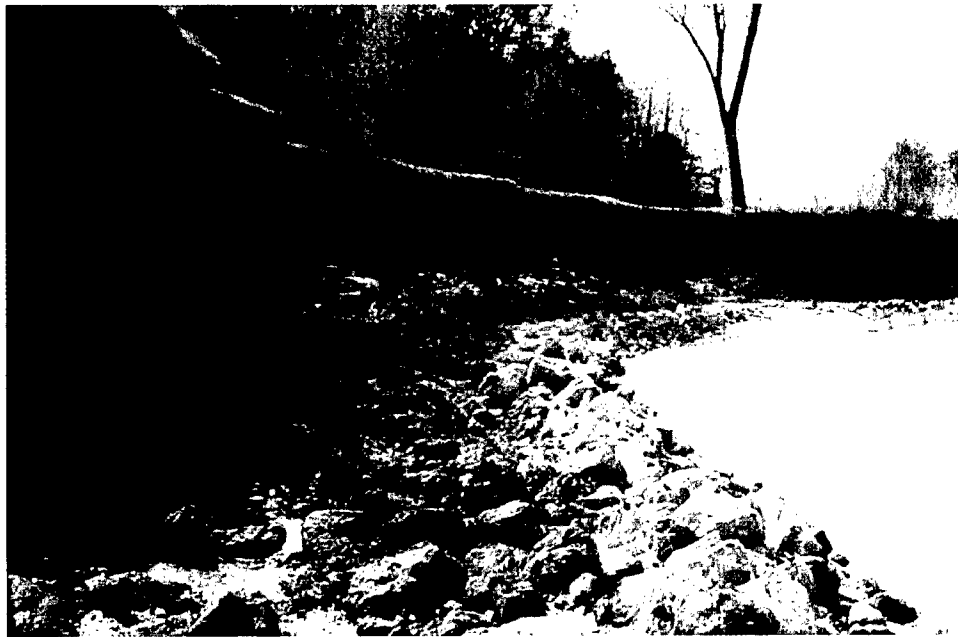
Figure 3. Bank stabilization with stone toe protection, Johnson Creek, MS
