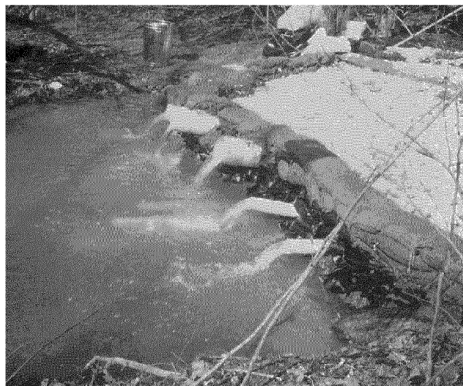
Figure 4-22. Sandbag underflow dam.
