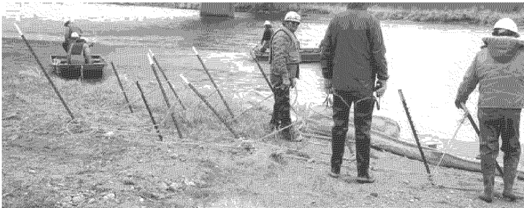
Figure 8-9. Multiple booms being anchored (DOWCAR, 1997).
