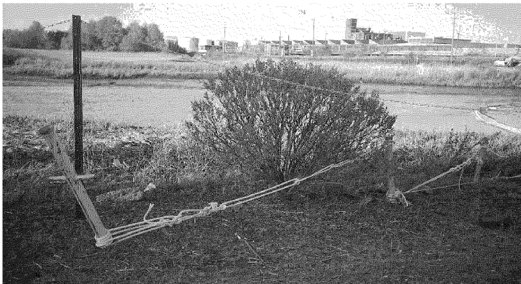
Figure 8-8. Multiple anchors used to moor boom.
