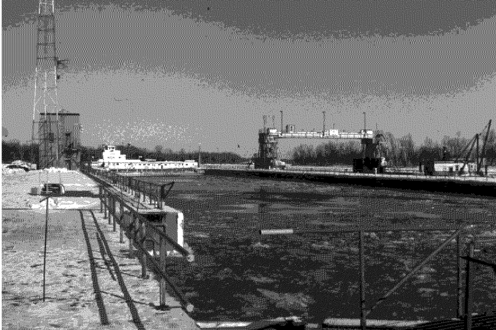
Figure 14. Le Grange Lock and Dam on the Illinois River. A free towboat washes brash ice from the upper approach, towards the submergible gate, adjacent to the lock chamber.
