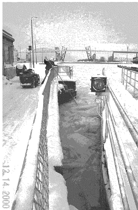
Figure 6. Clearing brash ice from the gate recess with a pike pole at the Soo Locks.
