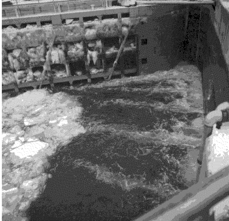
Figure 17. Gate recess flusher at Starved Rock Lock.
