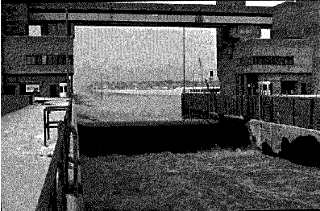
Figure 12. Submersible lift gate at Mel Price Lock.
