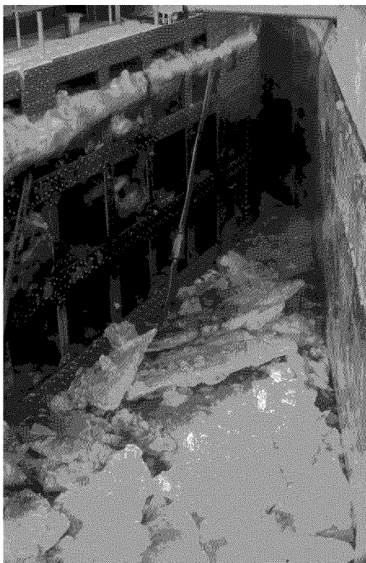
Figure 5. Brash ice in the miter gate recess.
