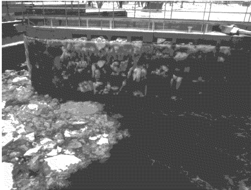
Figure 9. Icing of the miter gate trusswork.
