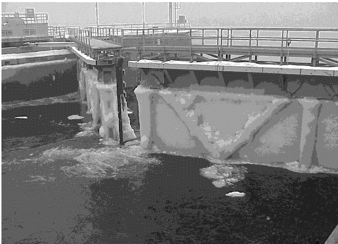
Figure 10. Miter at Lock 24 on the upper Mississippi with widely spaced structural members on the upstream side.
