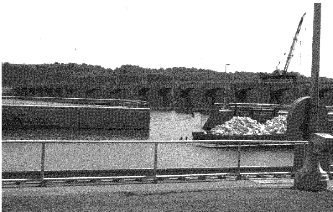
Figure 13. Drift pass in the river guardwall being widened at Lock and Dam 25 on the upper Mississippi.
