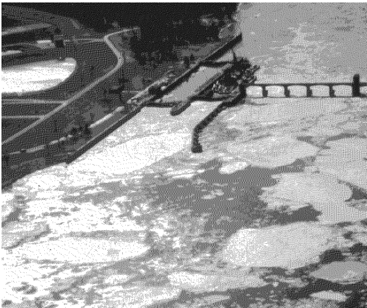
Figure 3. Ice accumulation in the upper approach at Lock and Dam 21 on the upper Mississippi River.
