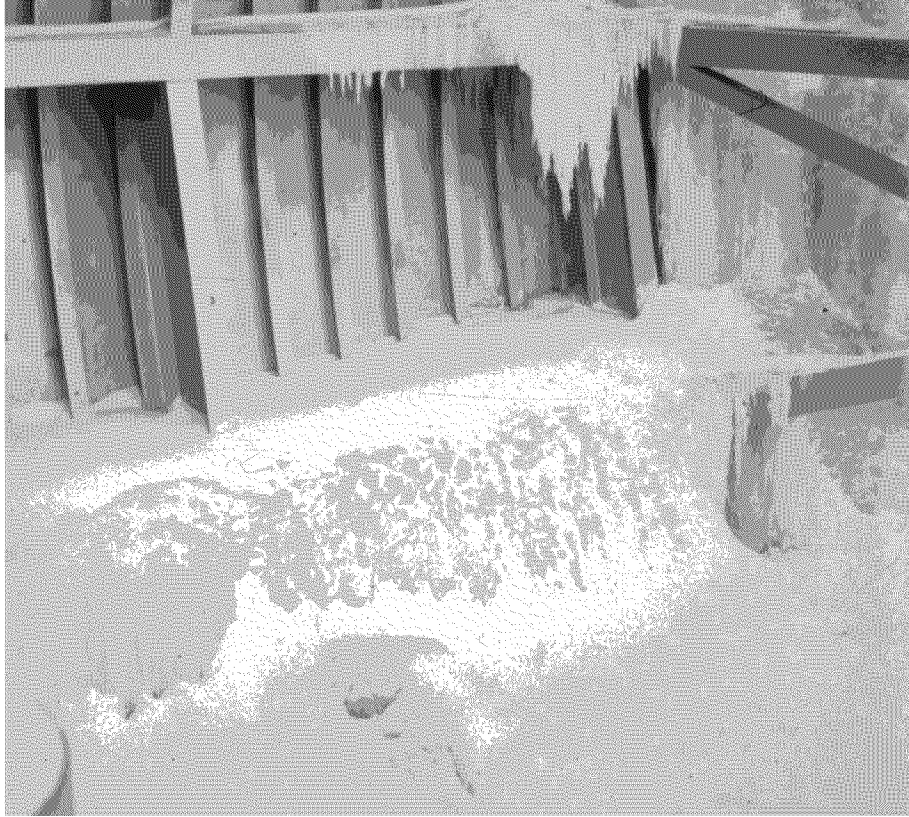
Figure 19. Iced-in tainter gate.
