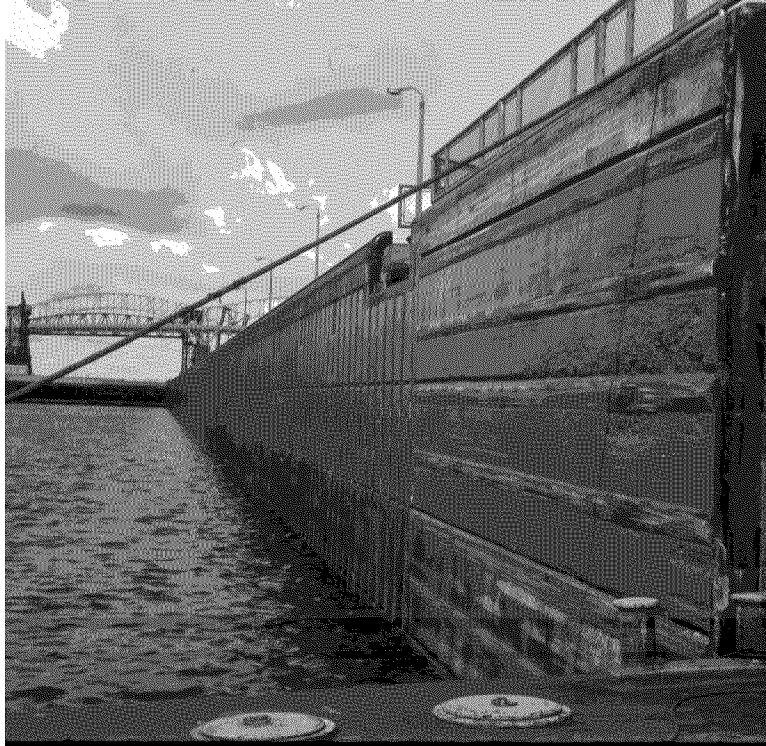
Figure 8. Copolymer coating at the Soo Locks.
