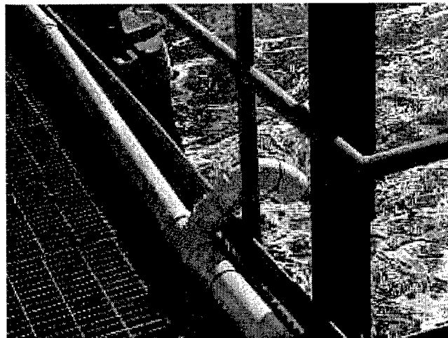
b. Access over the machinery access bridge
