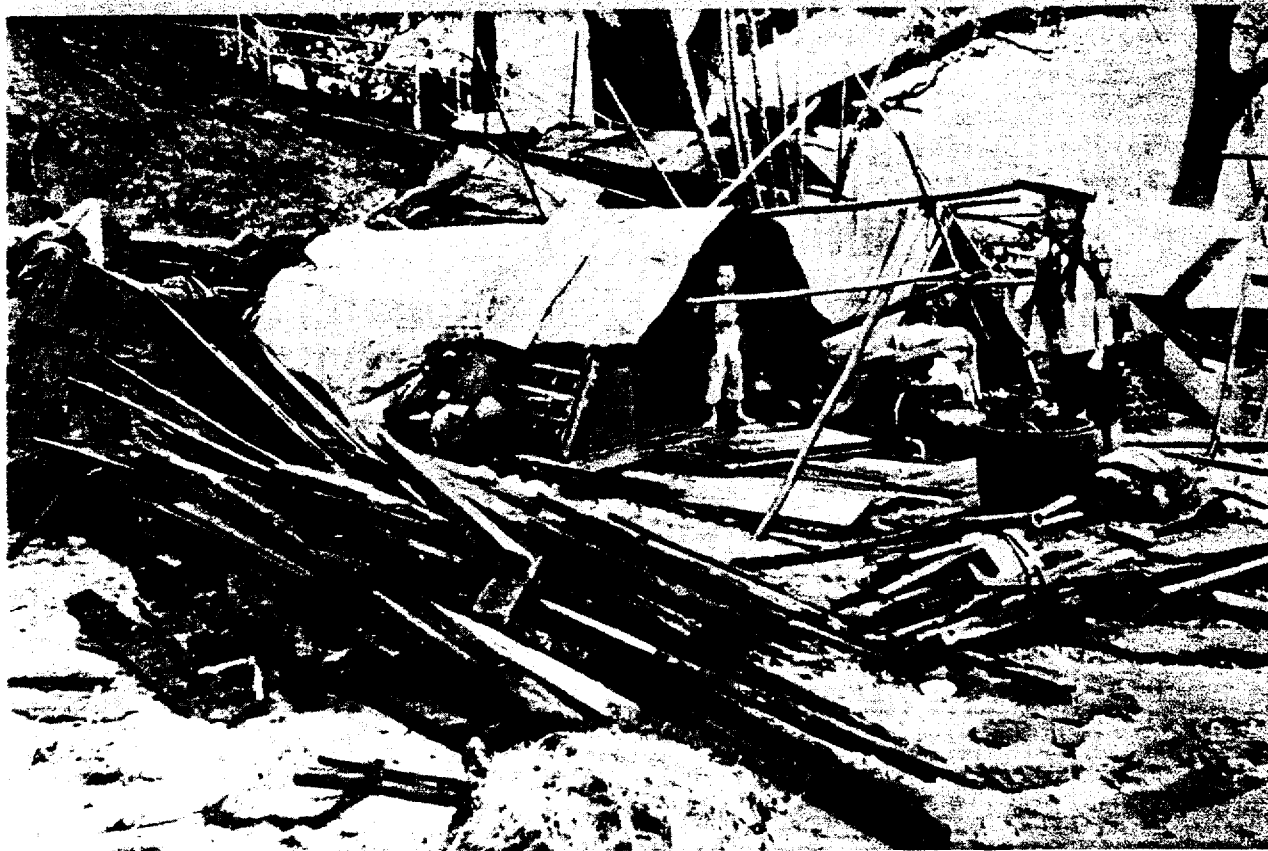
TYPHOON WANDA GUTTED TENEMENTS IN HONG KONG (TOP) AND LEFT CHILDREN ONLY MAKE-SHIFT DEBRIS OF A DAMAGED HOUSE (BOTTOM). (AP PHOTO)
