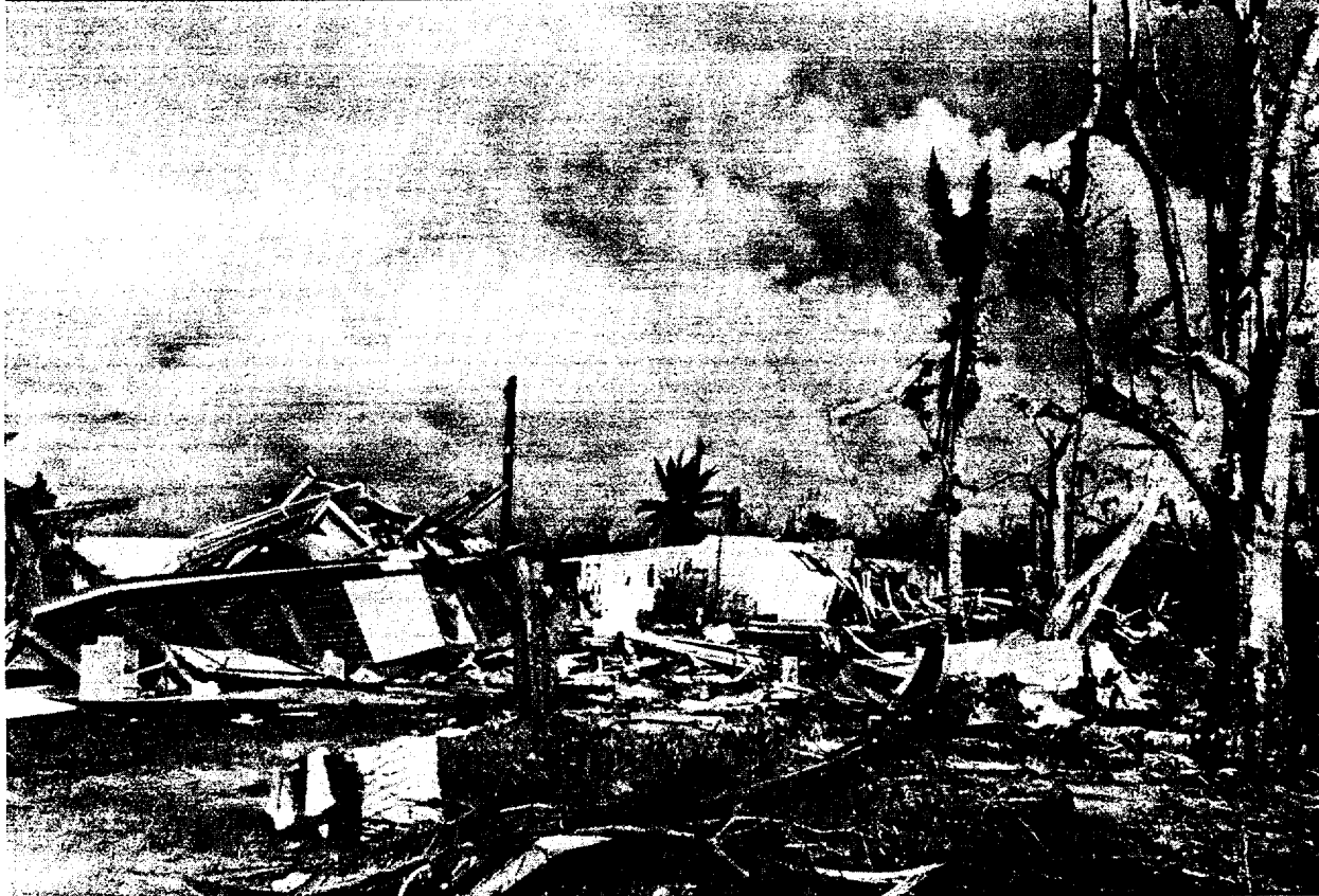
DEBRIS FROM WOODEN FRAME HOMES AND QUONSETS WAS STREWN OVER THE ISLAND OF GUAM BY TYPHOON KAREN. (USAF PHOTO)
