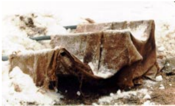
Figure 3. Cold-soaked burlap countermeasure.
